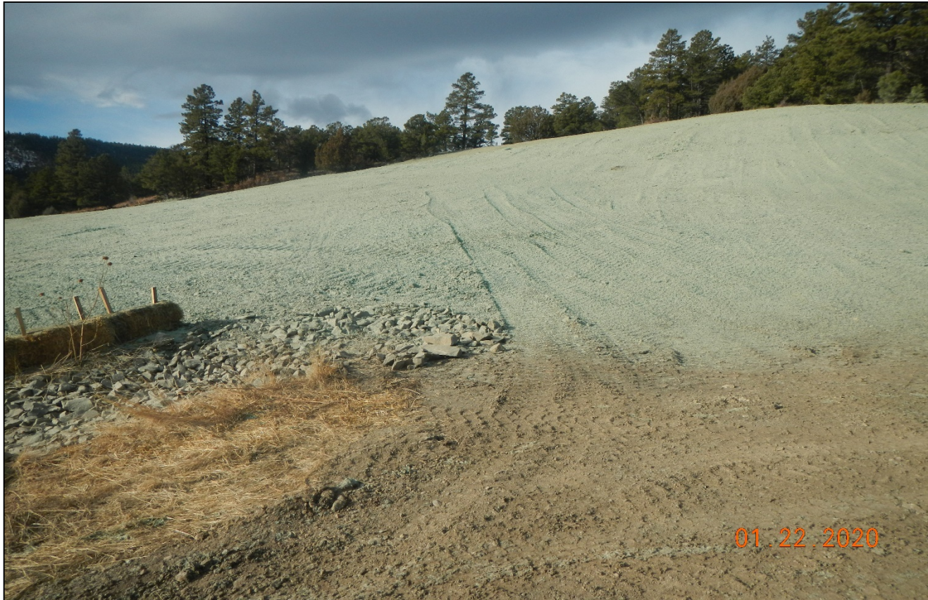
Photo 7. Facing southwest toward the top portion of the location where the cut slope was previously located. The location is recontoured and matches the surrounding contour of the terrain.
