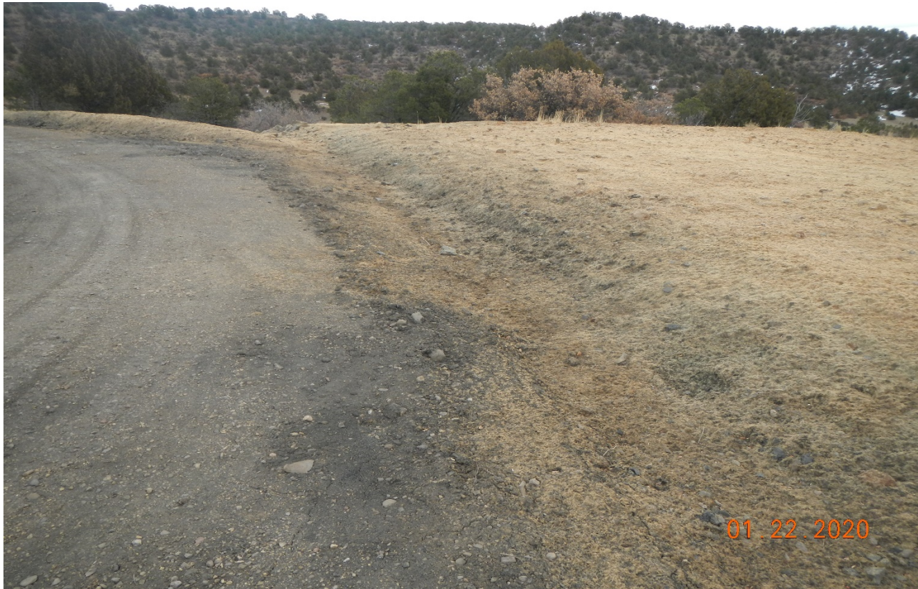
Photo 4. The south side of the location has been regraded, seeded, and hydromulched.
