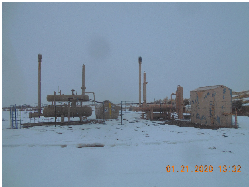
Separators with blowdown tank, Meter housing
