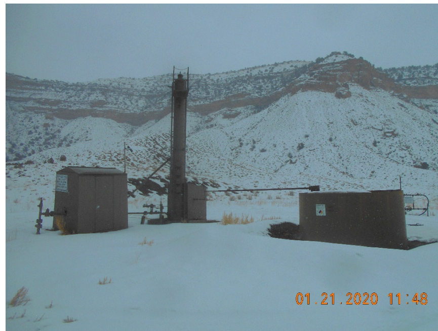
Meter housing, Dehydrator and Produced water tank
