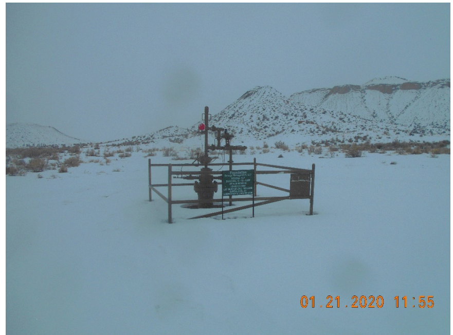
Wellhead with fence and sign
