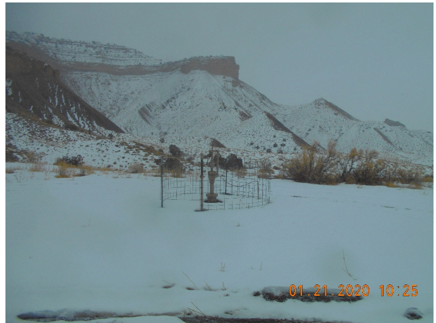
Wellhead with fencing.
