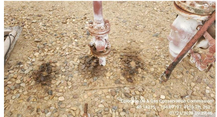
**Photo 7 Gas meter Runs Stained soil under flow line**
