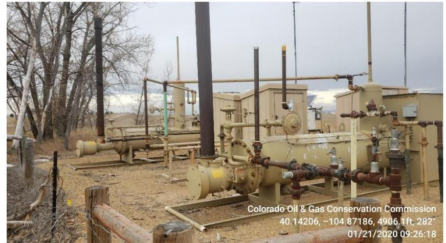
**Photo 5 ECDs, Gas Meter Run & Horiz. Heated Separator**
