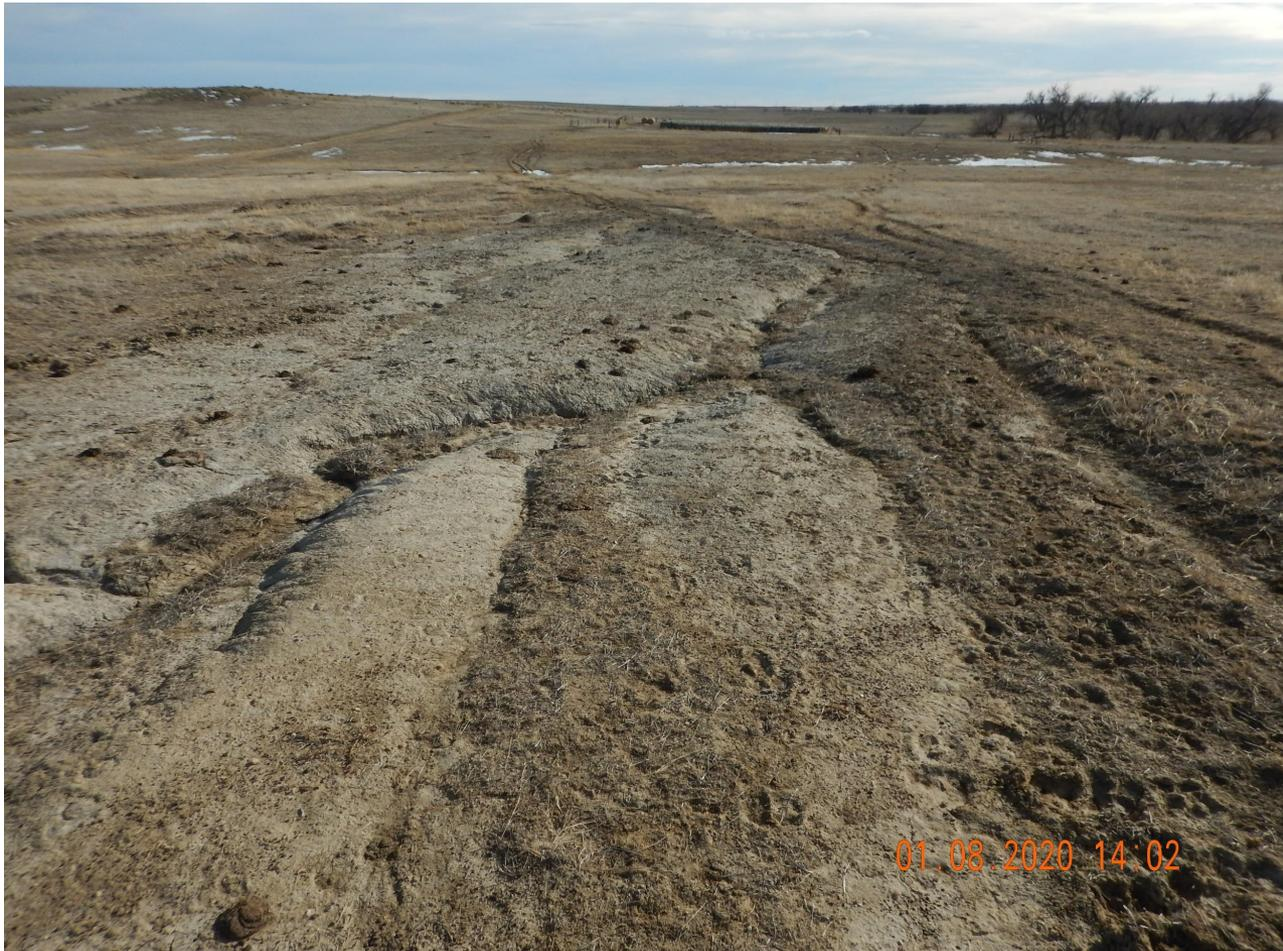
**Photo 7.** Photo taken from the southern tank battery, facing South. Photo illustrates erosion occurring along portions of the produced water spill.
