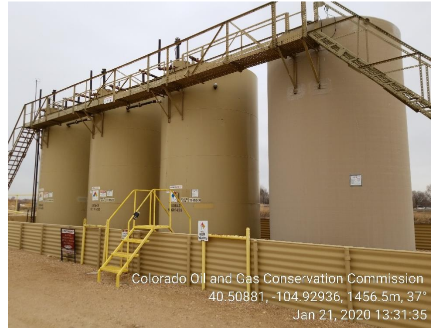
Photo 4: Tank Battery
