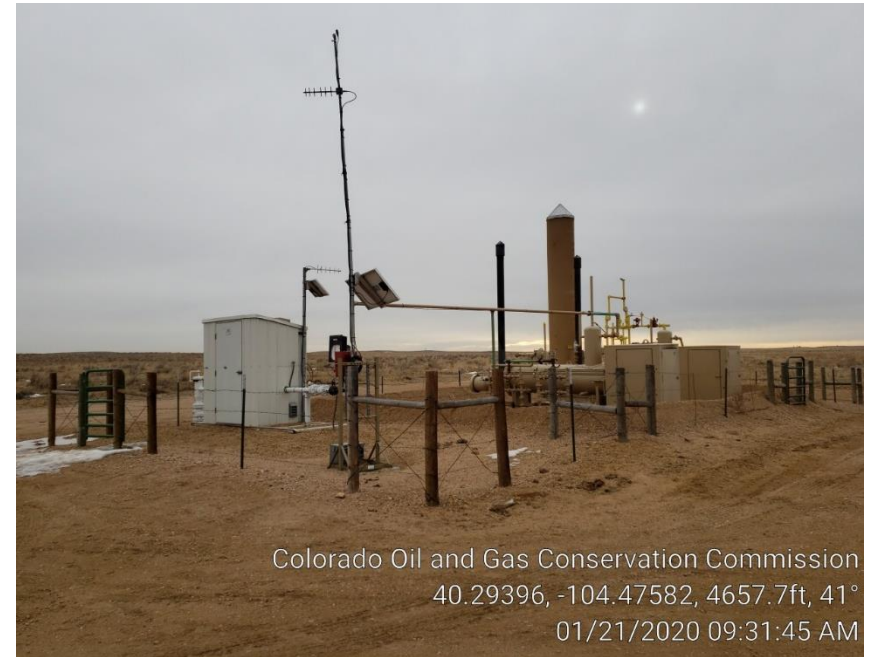
Photo #2 Separator's, ECD & Meter Run
