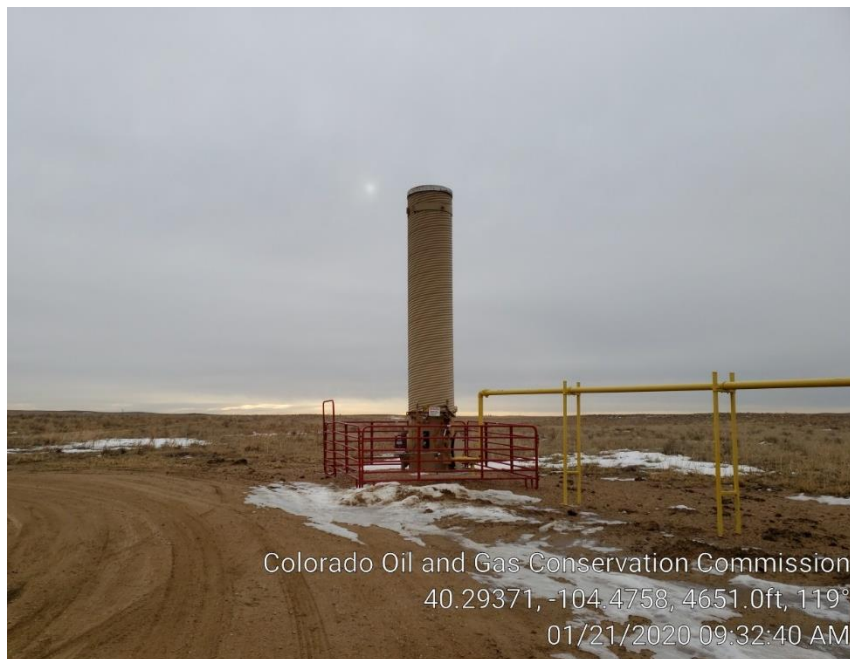
Photo #3 ECD for production tanks
