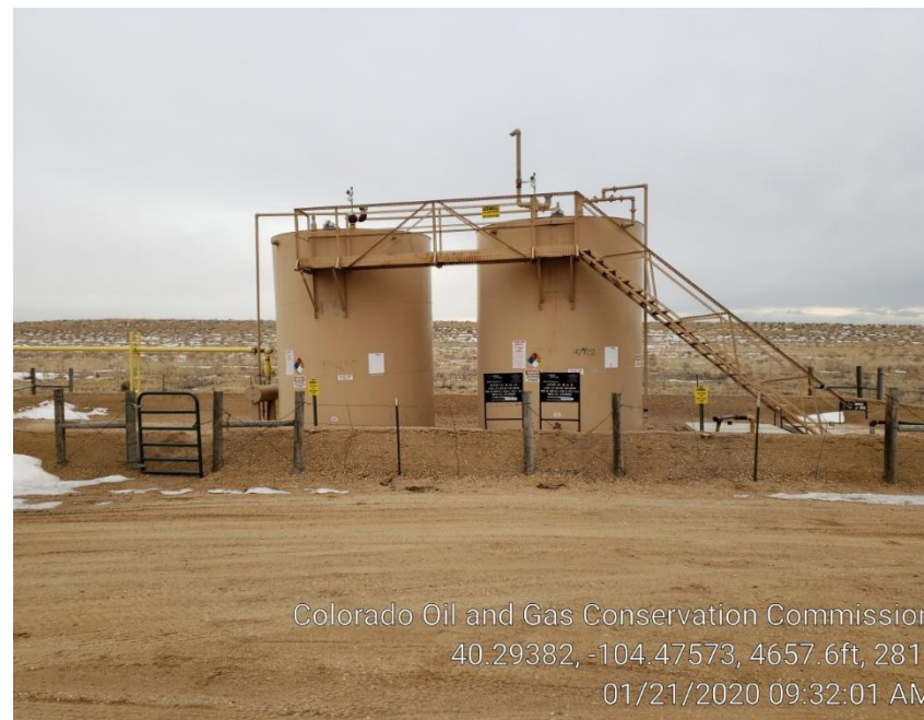
Photo #4 Tank Battery
