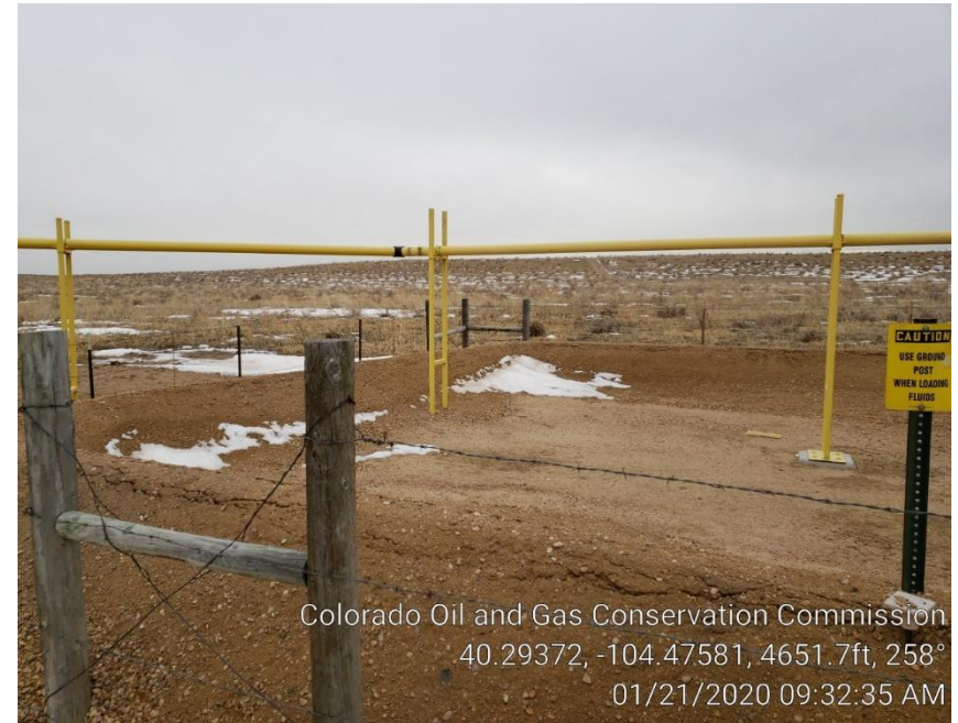
Photo #6 Repaired Berm
