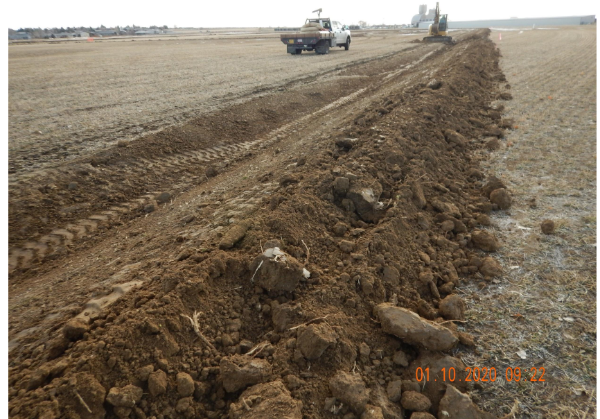
Photo 2. Photo taken from the Southwestern perimeter of location on January 10, 2020, facing East. Photo illustrates a ditch and berm BMP in the foreground. In the background sediment trap BMPs installation.
