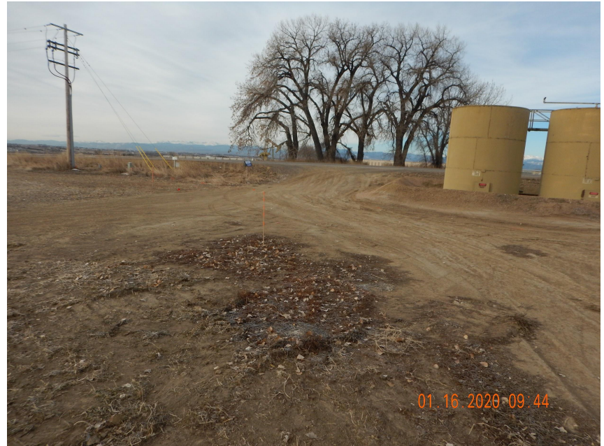
Photo 11. Photo taken from the entrance of location on January 16, 2020, facing West. Photo illustrates that entrance has pre-existing gravel. Operator will likely be required to install additional tracking device BMPs once more equipment is mobilized to location.
