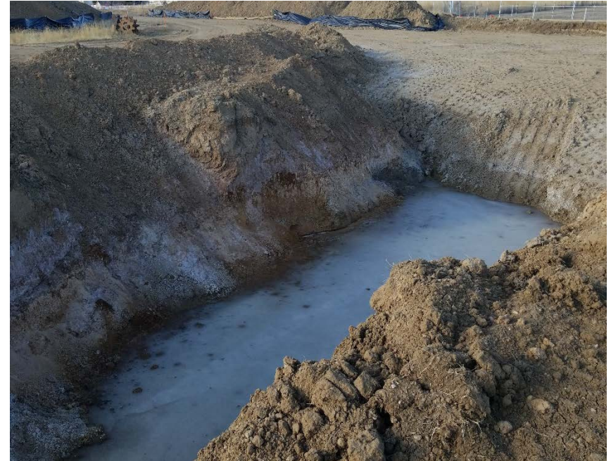
Photo 6: Portion of the open excavation being infiltrated by ground water.
