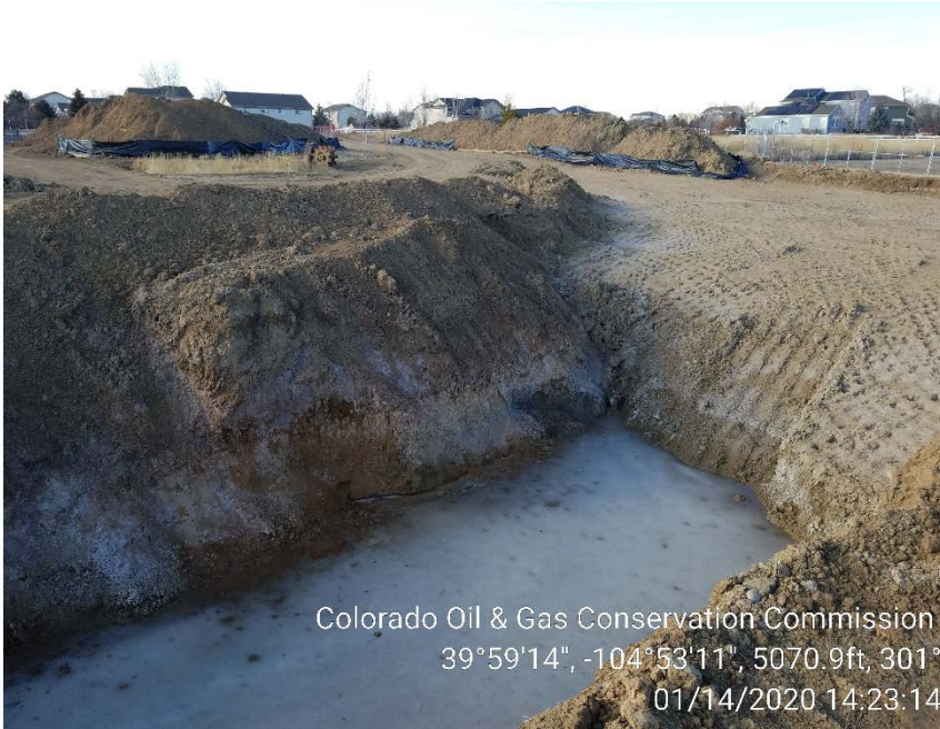
Photo 5: Portion of the open excavation being infiltrated by ground water.
