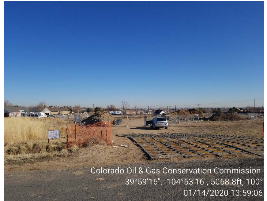
Photo 2: Tracking pad at gate in the perimeter fence.
