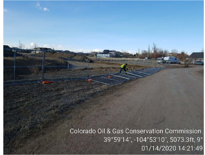
Photo 4: Repairs to portion of the perimeter fence that blew down.
