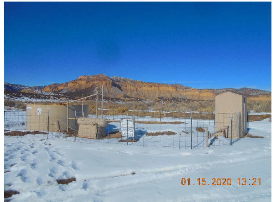
Separator, Meter housing, Produced water tank and Pit #119477 with fence and sign.
