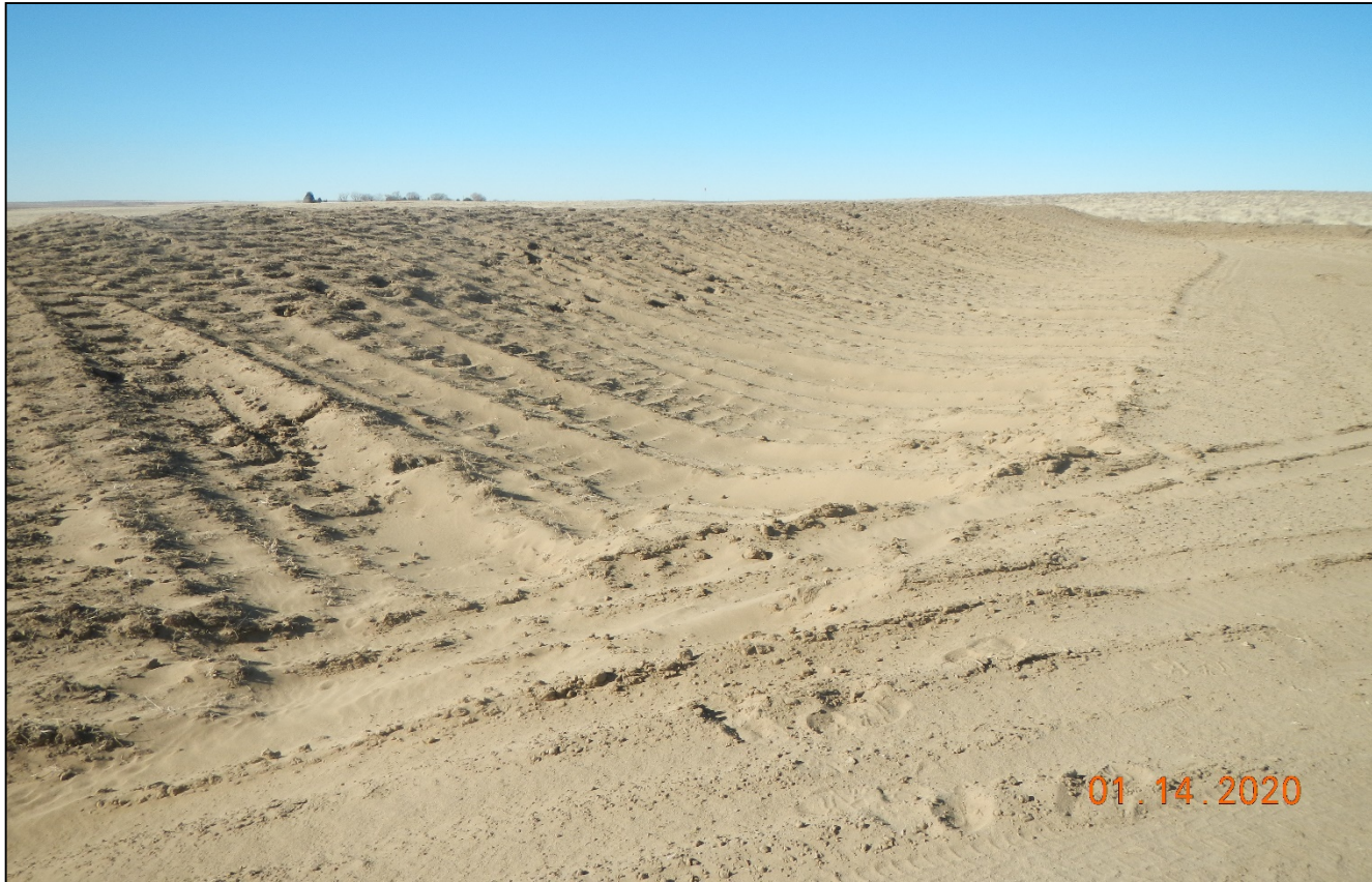
Photo 4. Topsoil pile at west side of the location has been tracked in. The soils are sandy and susceptible to wind erosion. Additional BMP's will be needed for stabilization.
