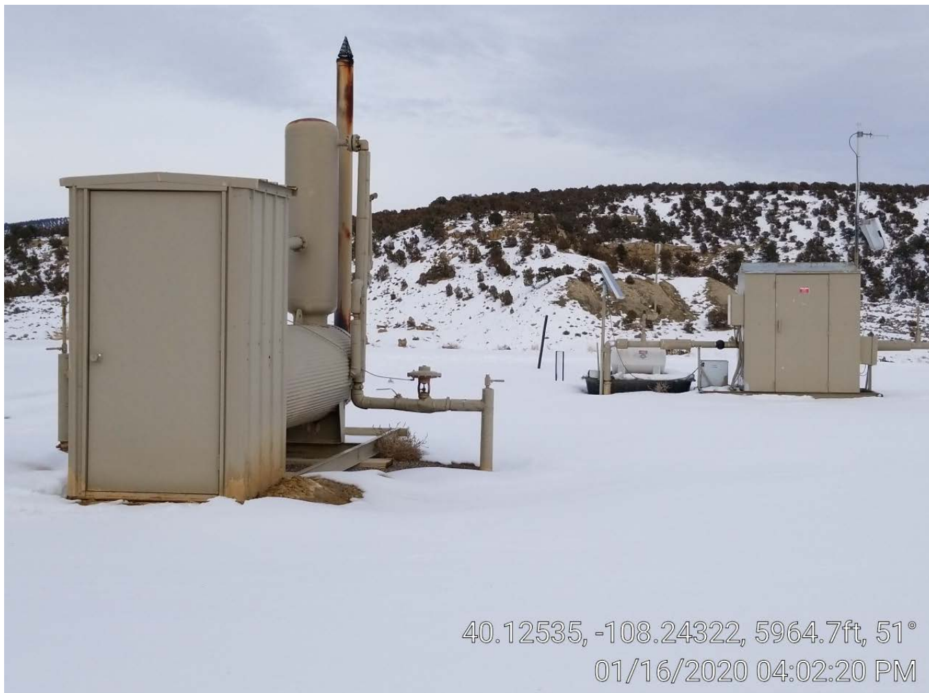
Photo 3. Separator & meter building.
