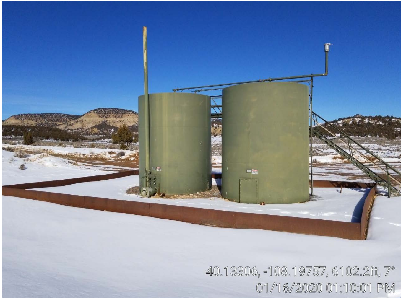
Photo 4. Tank battery.
