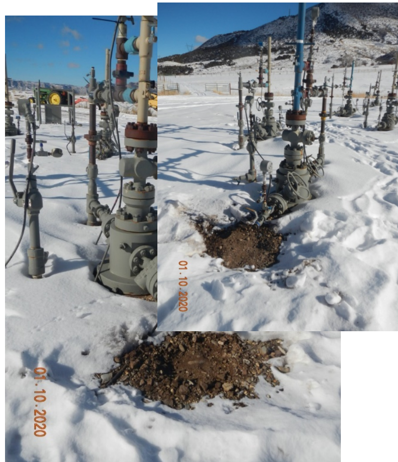
Photo#7: Drip areas at Wellheads.
