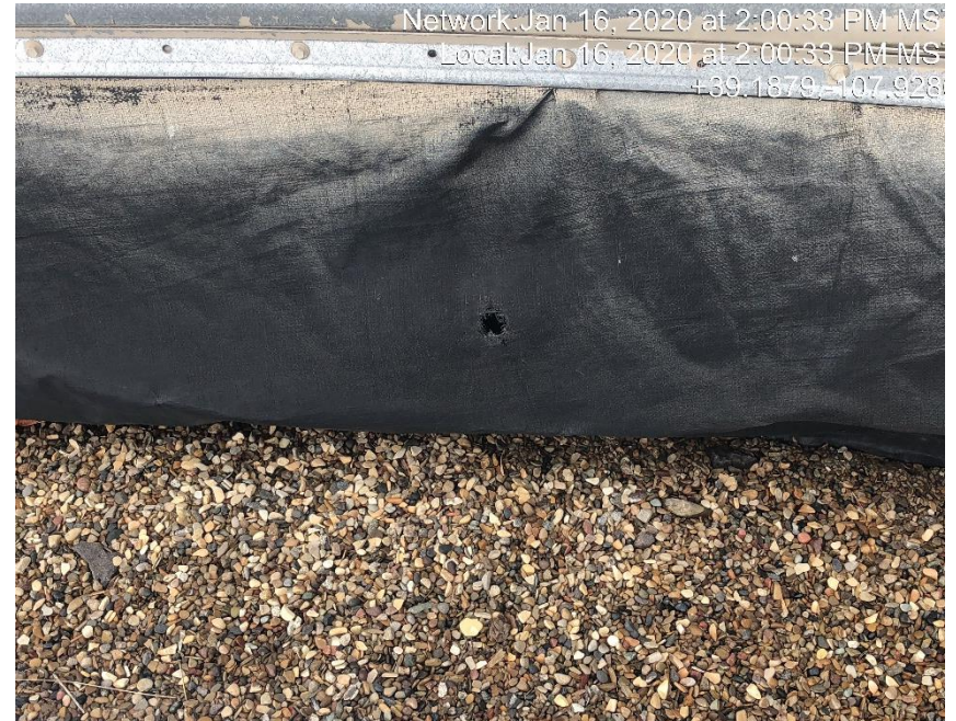
Photo #0431 Hole in tank containment liner.
