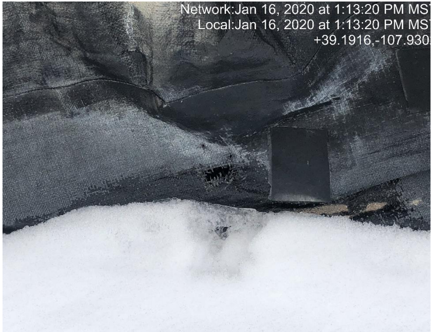
Photo #0429 Multiple holes in tank containment liner.
