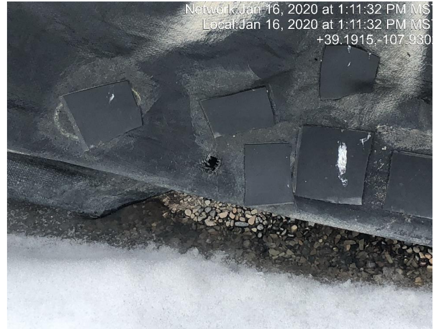
Photo #0425 Multiple holes in tank containment liner.
