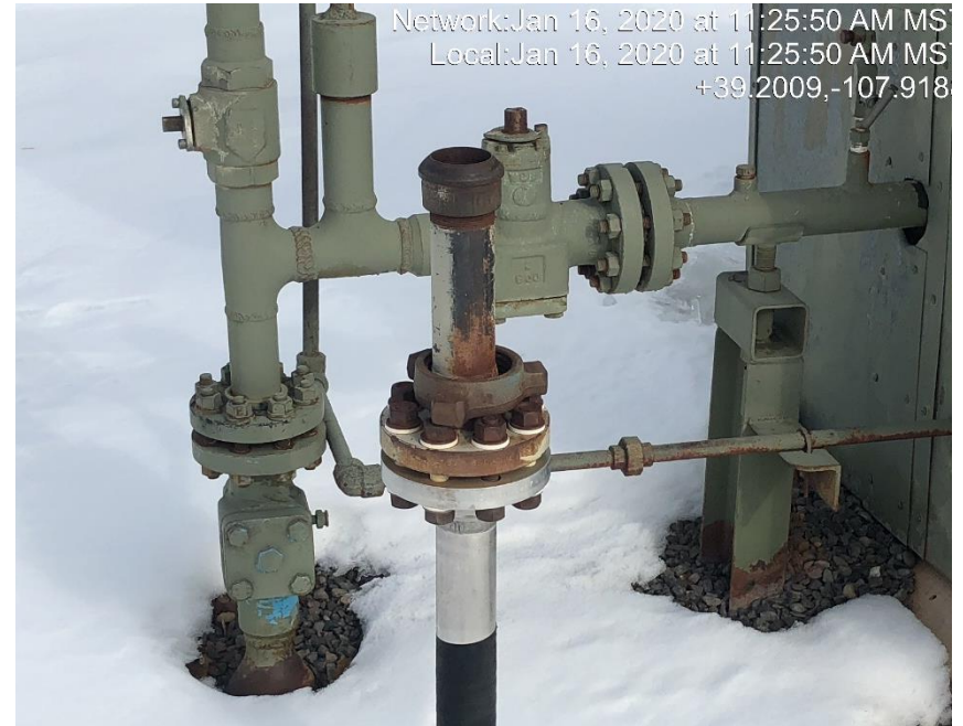
Photo #0422 Flowline riser by meter run not LO/TO.
