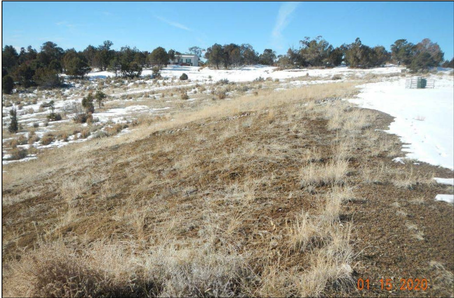
Photo 2. View of the southern fill slope from the southeastern corner facing westward. Based on operator submitted documentation, re-seeding was conducted in 2018. As vegetation is in a dormant condition, germination and revegetation success should be assessed during the active 2020 growing season.
