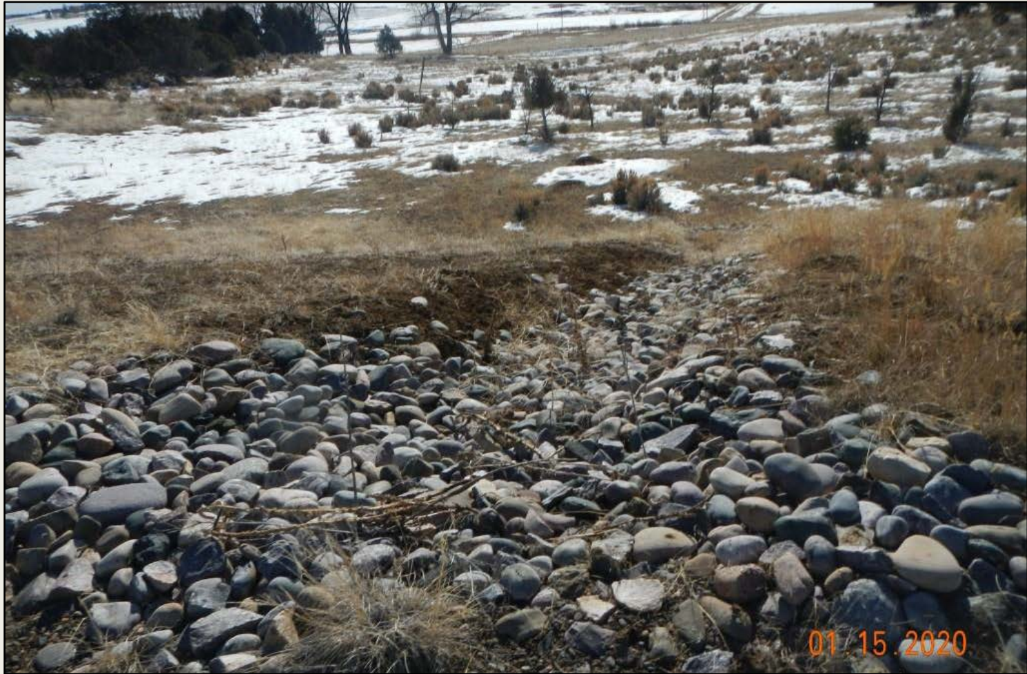
Photo 4. View of cobble run-down placed in the southern project area. Operator should note that cobble rock is not considered a BMP, as it does not effectively reduce energy of stormwater flows. Course rock is needed where rock is used as a stormwater BMP. Operator needs to continue to monitor stormwater erosion and apply BMPs according to good engineering practices when/where stabilization is needed.
