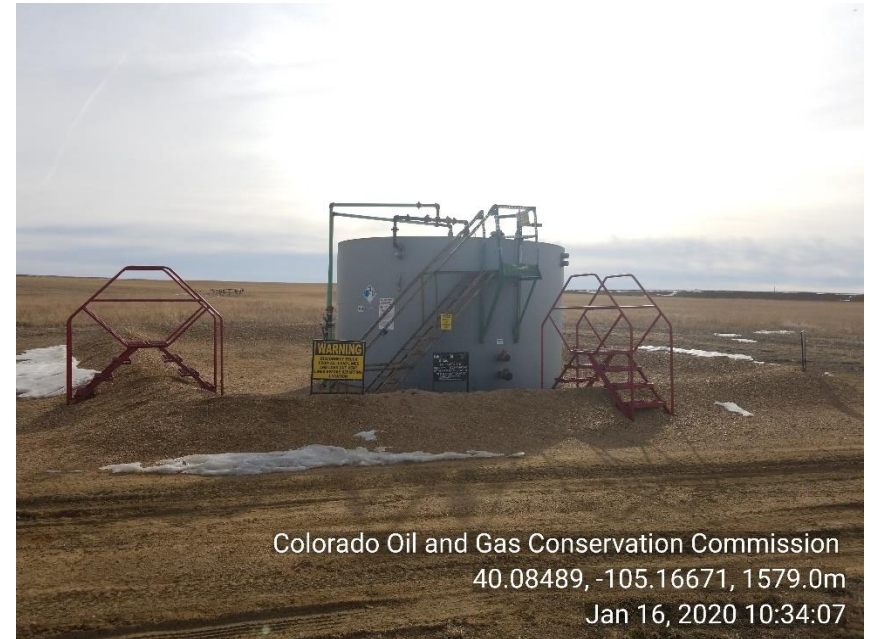
Photo 4 TNK BTRY. Facility paint not uniform (crude oil tank)
