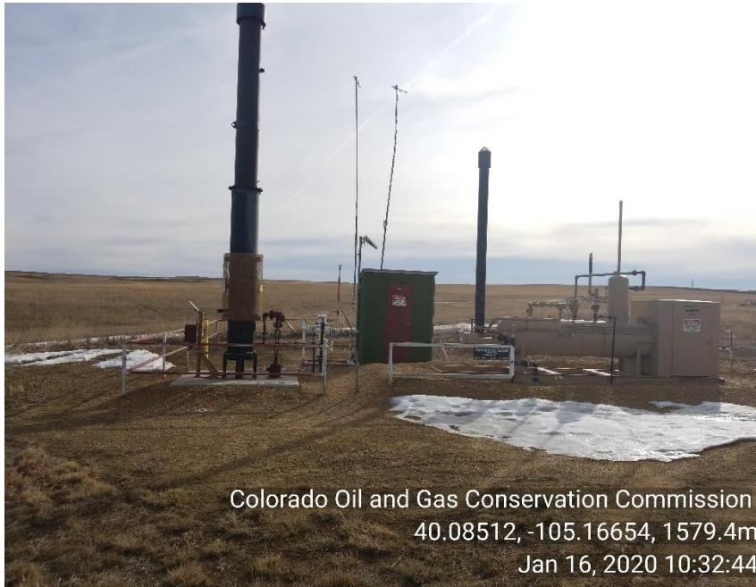
Photo 3 Sep/meter house and ECD. Facility paint not uniform (meter house).
