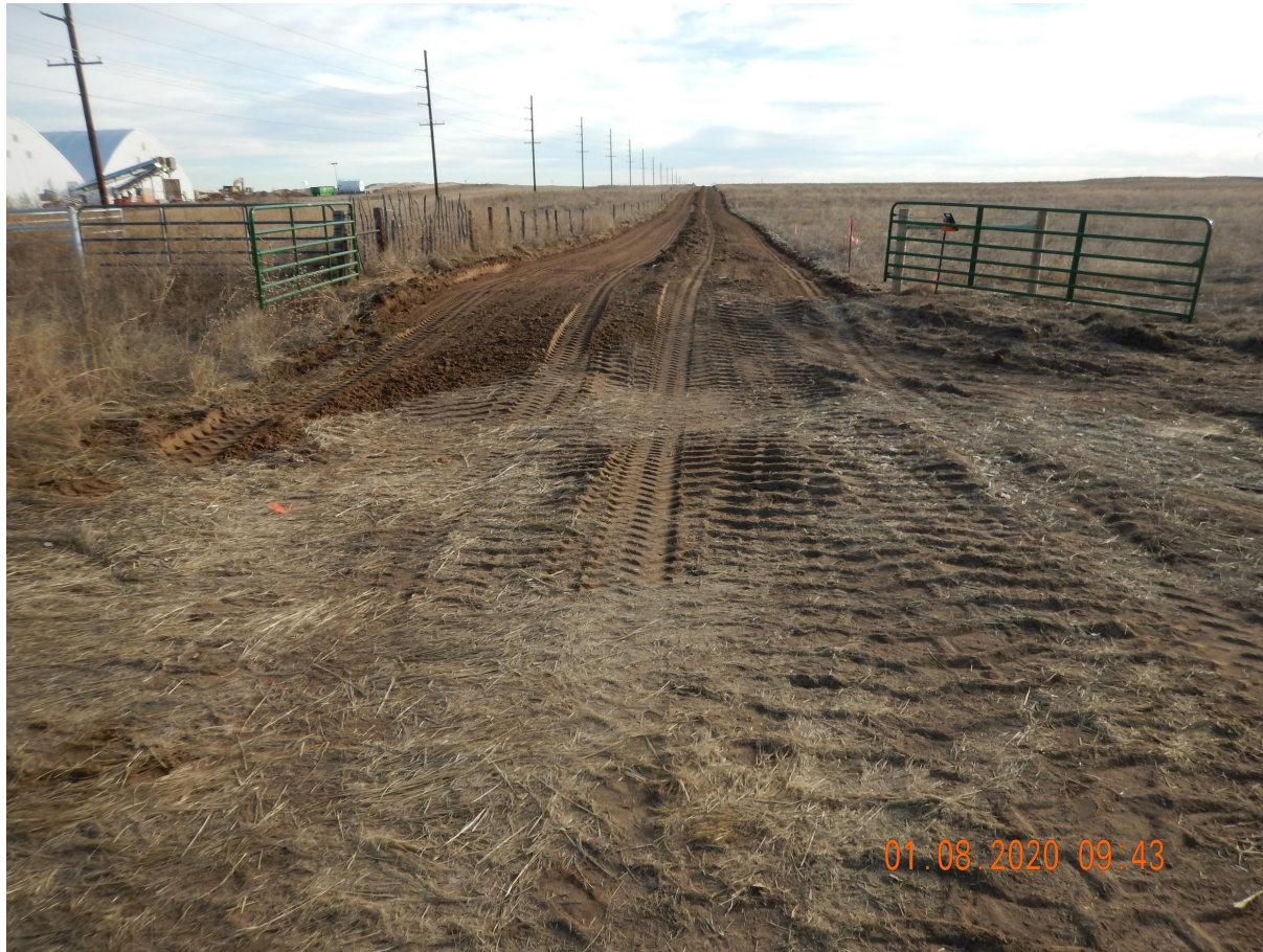
Photo 1. Photo taken from the entrance of location, facing East. Photo illustrates Operator has not yet installed vehicle tracking device BMPs. Operator should consider installing this as one of the first BMPs.
