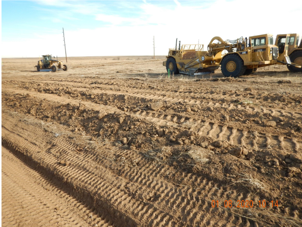
Photo 3. Photo taken from the western perimeter of location, facing Northeast. Photo illustrates topsoil is being salvaged and stored along the western perimeter of location.
