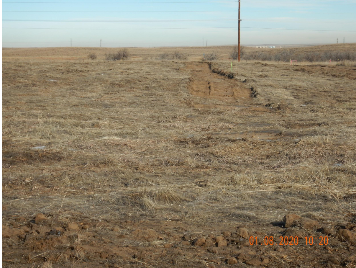
Photo 7. Photo taken from the southern perimeter of location, facing North. Photo illustrates Operator is in-process of performing topsoil salvage operations.
