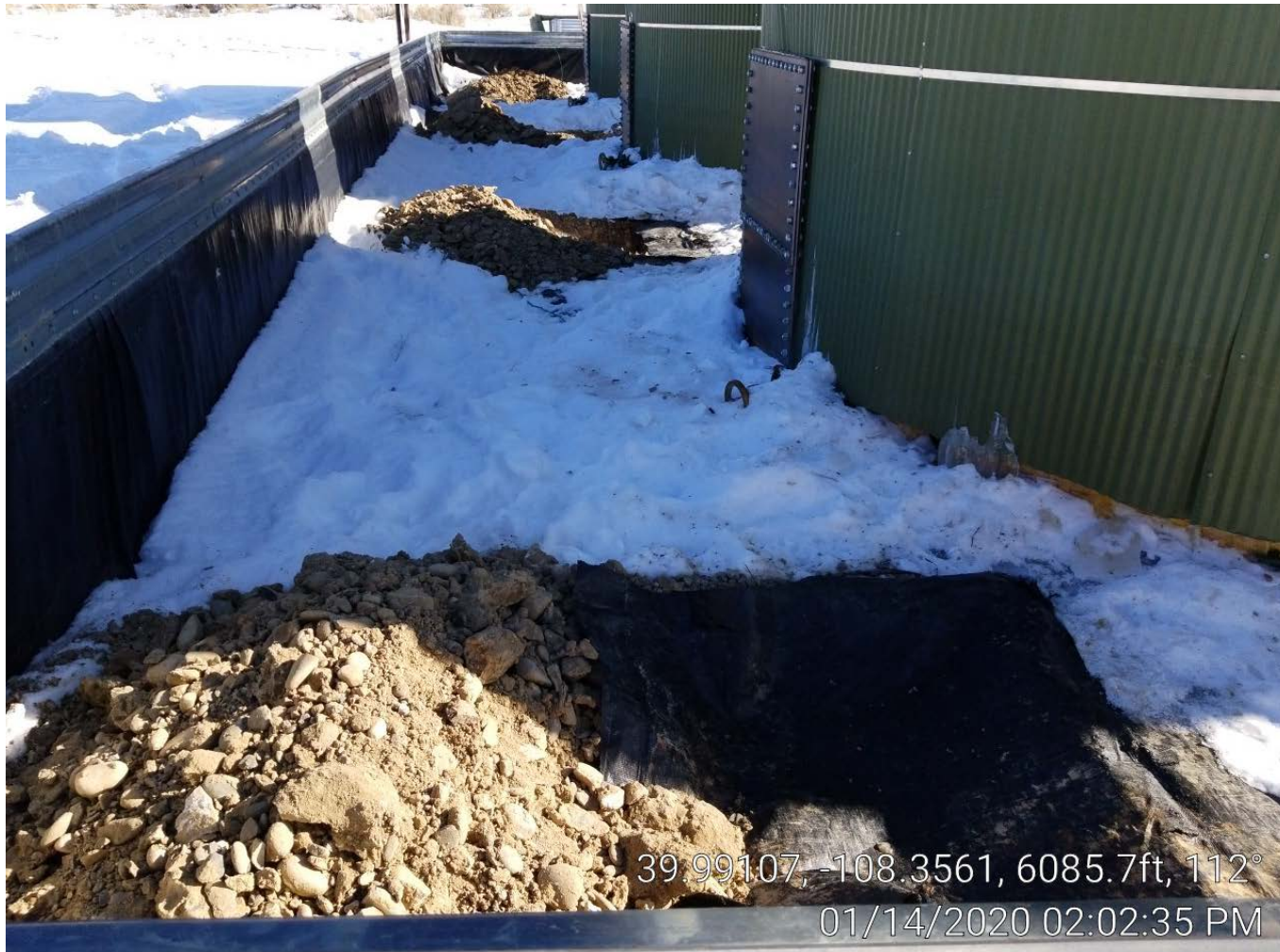
Photo 5. Secondary containment excavations.
