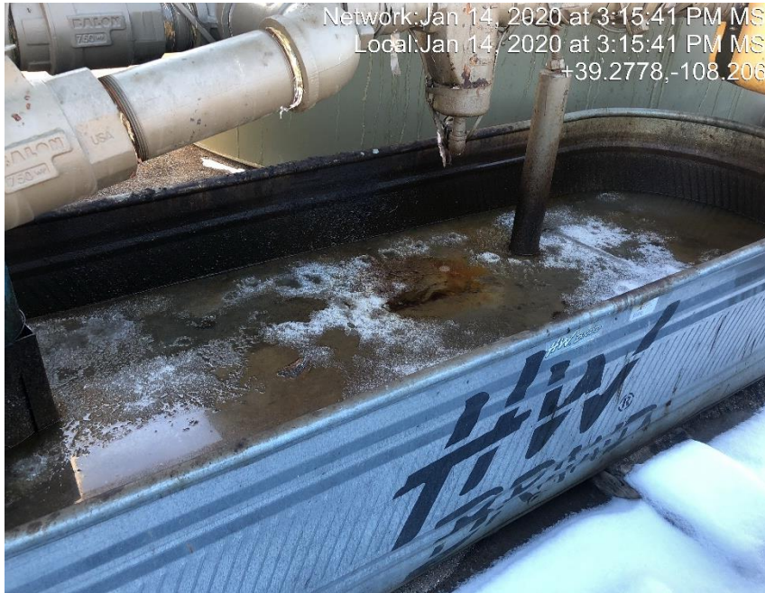
Photo #0412 Oily fluid in stock tank inside tank containment.
