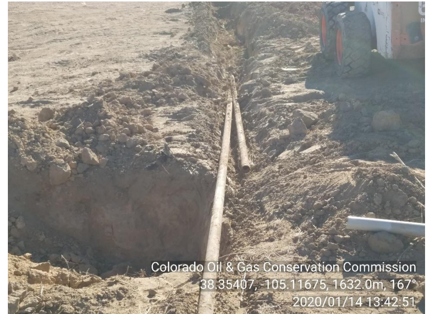
PHOTO 4: flow lines being removed
