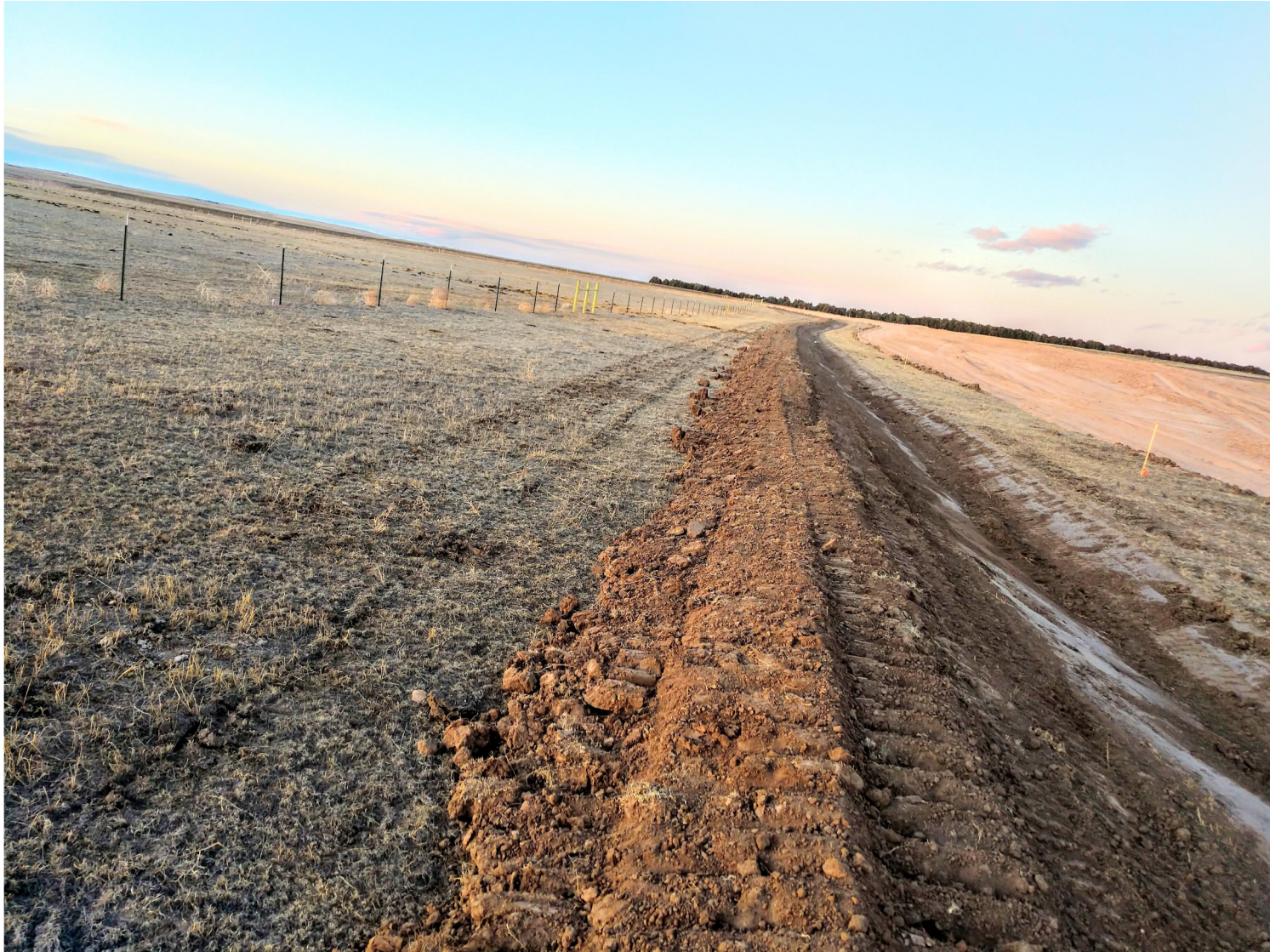
Western edge Perimeter Ditch – looking North – Berm has been compacted
