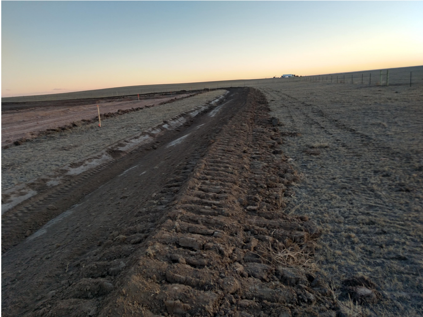
Western edge Perimeter Ditch – looking South – Berm has been compacted
