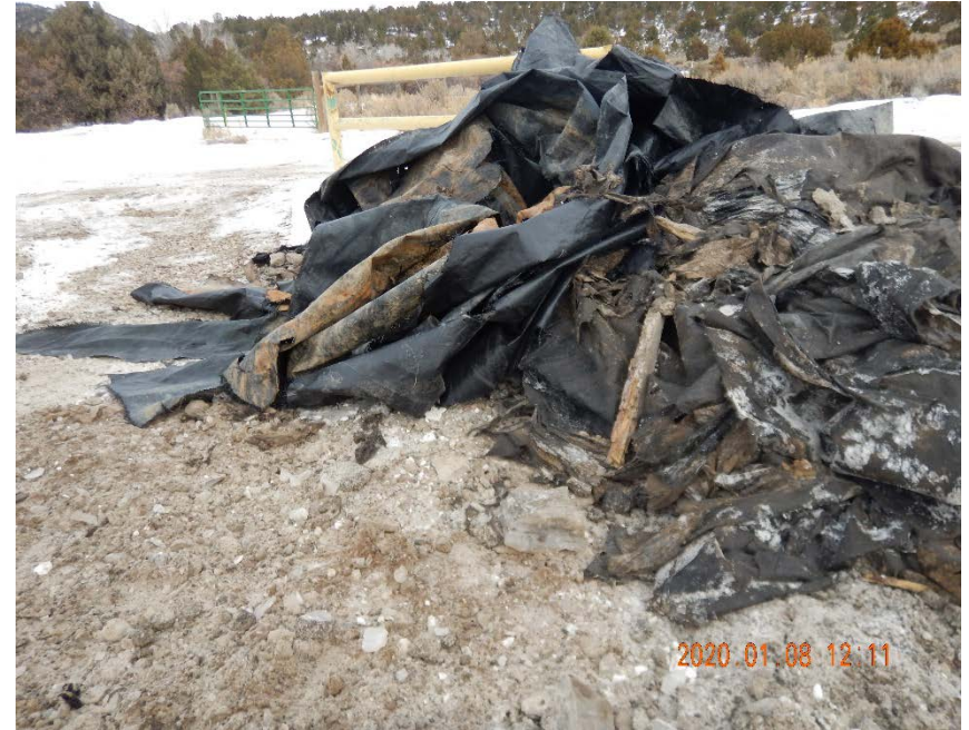
Photo #6 - Tank battery liner material and felt remaining on east side of former north tank battery area.
