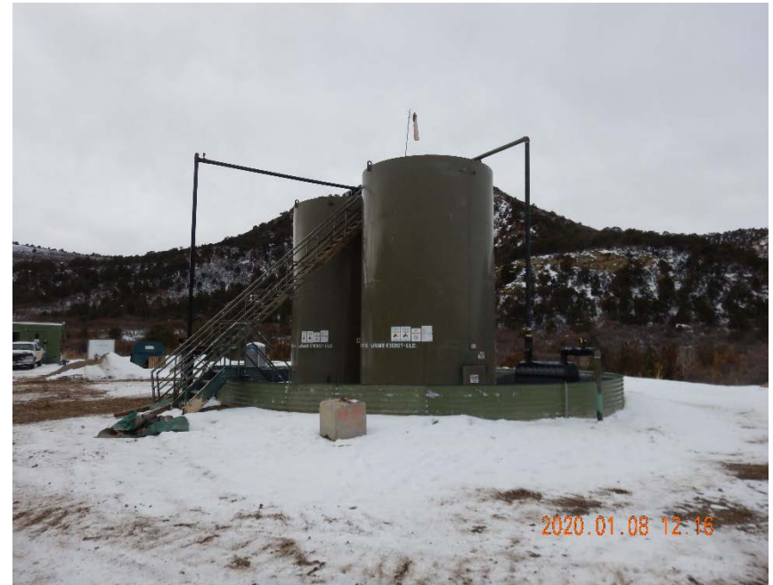
Photo #12 – View of two (2) 400 bbl steel ASTs labeled to contain both condensate and produced water located inside of lined, metal secondary containment at northwest side of pad. Northwest tank battery.
