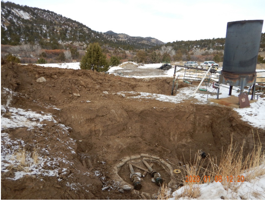
Photo #9 – Additional exposed flowlines inside of excavation in ECD area.
