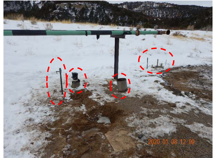
Photo #4 – Uncapped and capped flowlines and flowline risers as well as cement debris, bucket, and felt/liner scraps remaining in former north tank battery area.
