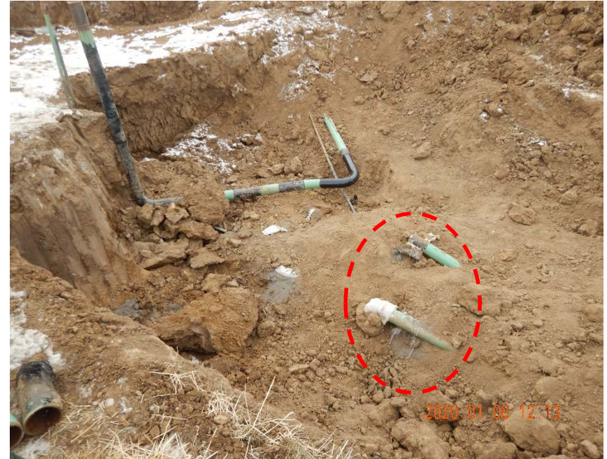
Photo #8 – View of flowlines inside of open excavation inside ECD area . Note red circle marks the location of two cut flowlines.
