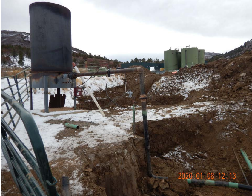
Photo #7 – ECD area , exposed flowlines, and open excavations remain south of former tank battery area.
