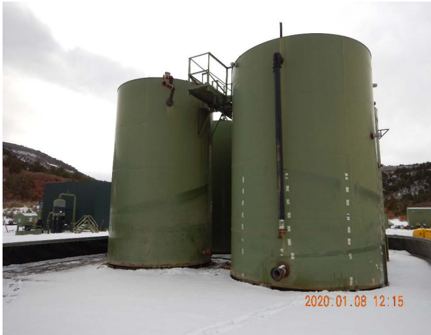
Photo #11 – View of four (4) 400 bbl steel ASTs labeled “Produced Water” located inside of lined, metal secondary containment in center of pad. Central tank battery.
