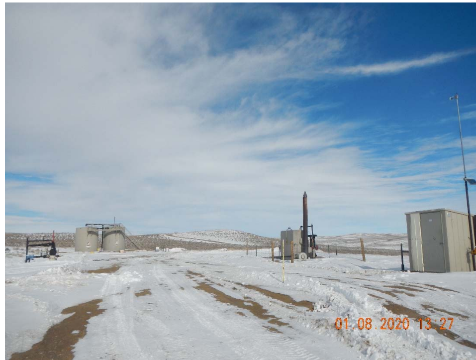
Photo 1. Overview of location taken facing north.
