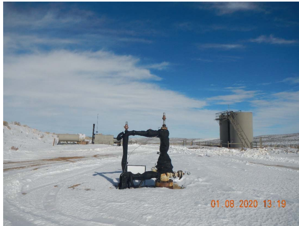
Photo 1. Overview of location taken facing north.
