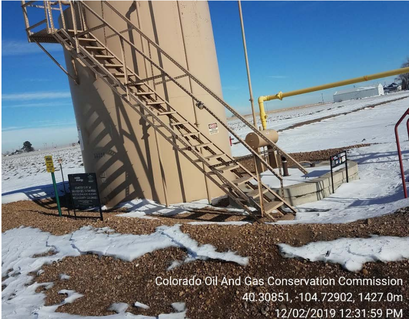
Crude oil tank berm on 12/2/2019
