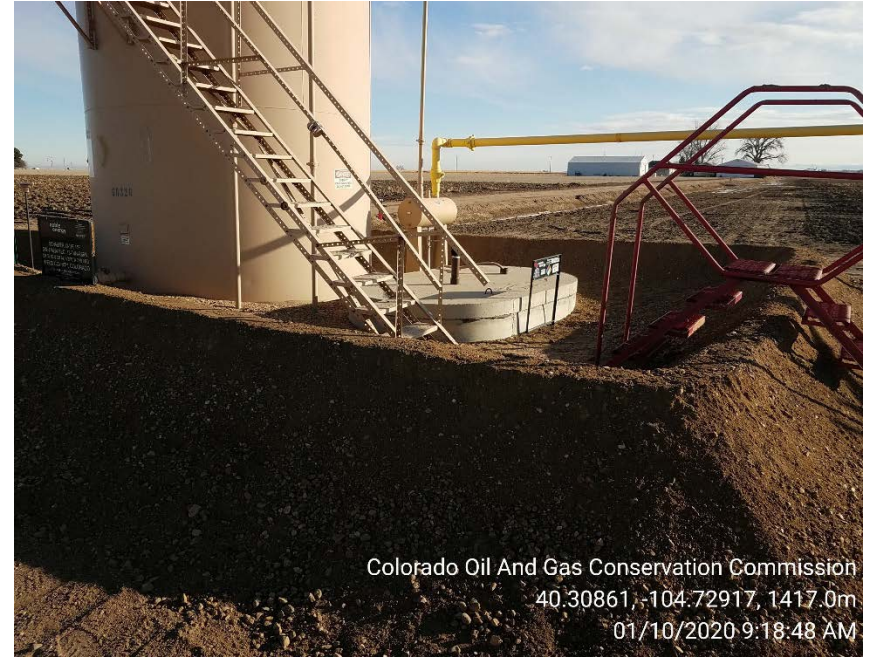
Crude oil tank berm on 1/10/2020
