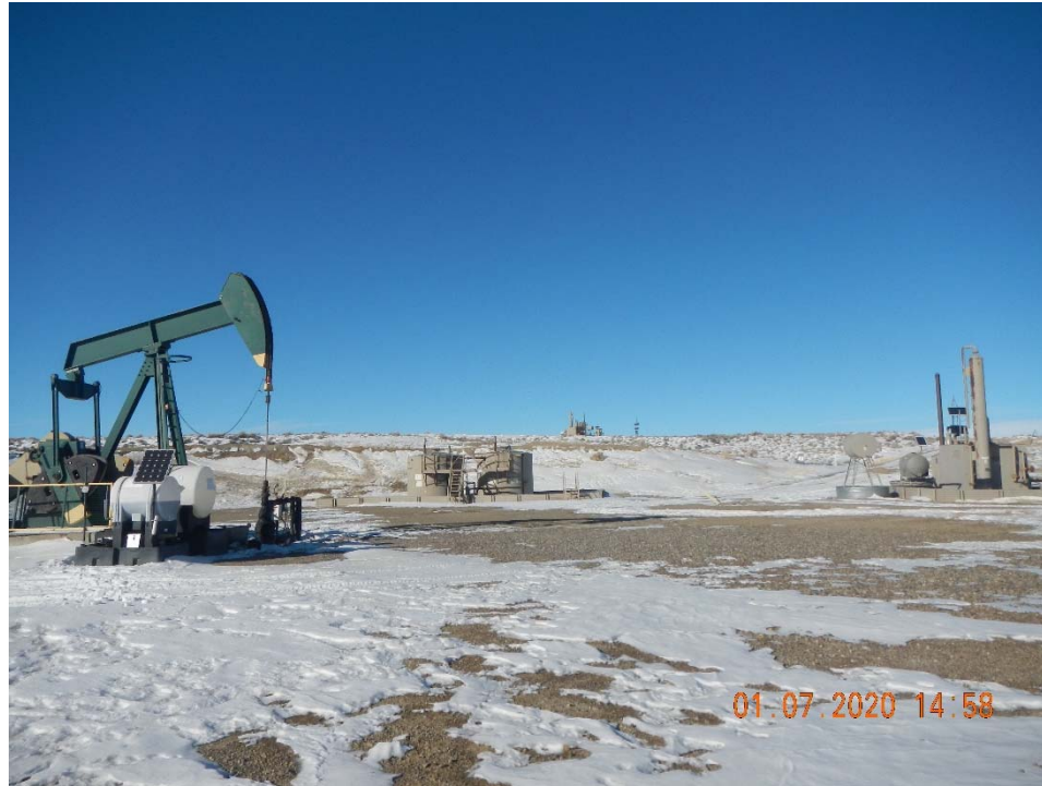
Photo 1. Overview of location taken facing north.
