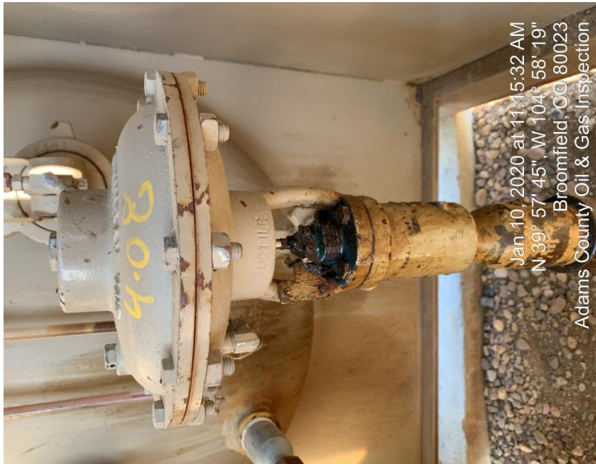
Photo#3 Corrective Action:Oil dump leaking
