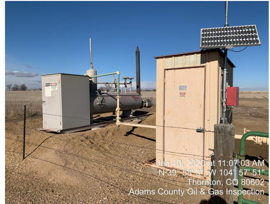
Photo#2 Gas Meter/Separator/Automation RTU
