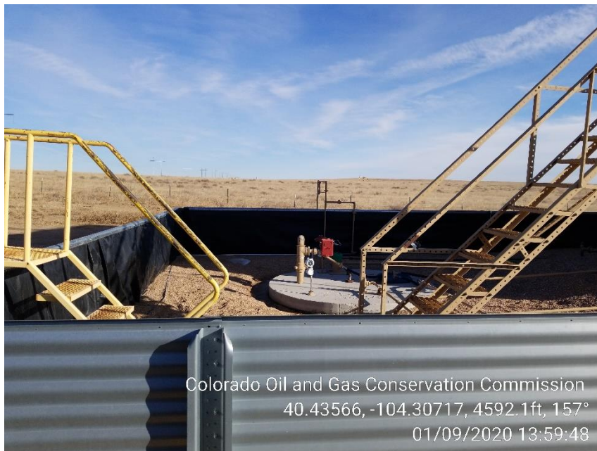
Photo 3 – 60 BBLS Concrete vault is missing Content and Capacity Labels
