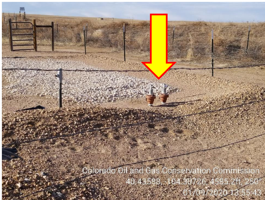
Photo 5 – Unmarked Risers
