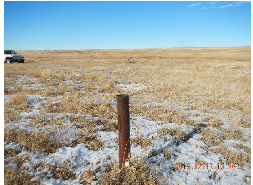
Photo 6: Open ended riser (2) of (2).
