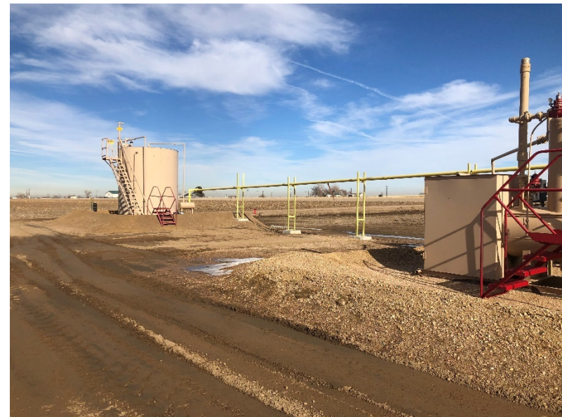
Photo NBL2. Production facility, facing northeast. Secondary containment has been repaired to provide adequate containment per 605.a.(4).
