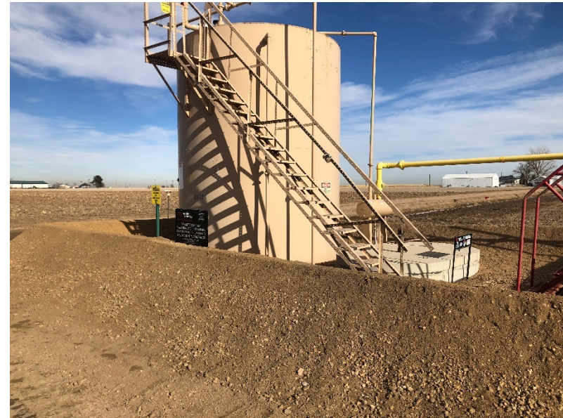
Photo NBL3. Berm surrounding crude oil tank and produced water pit, facing northeast. Secondary containment has been repaired to provide adequate containment per 605.a.(4).
