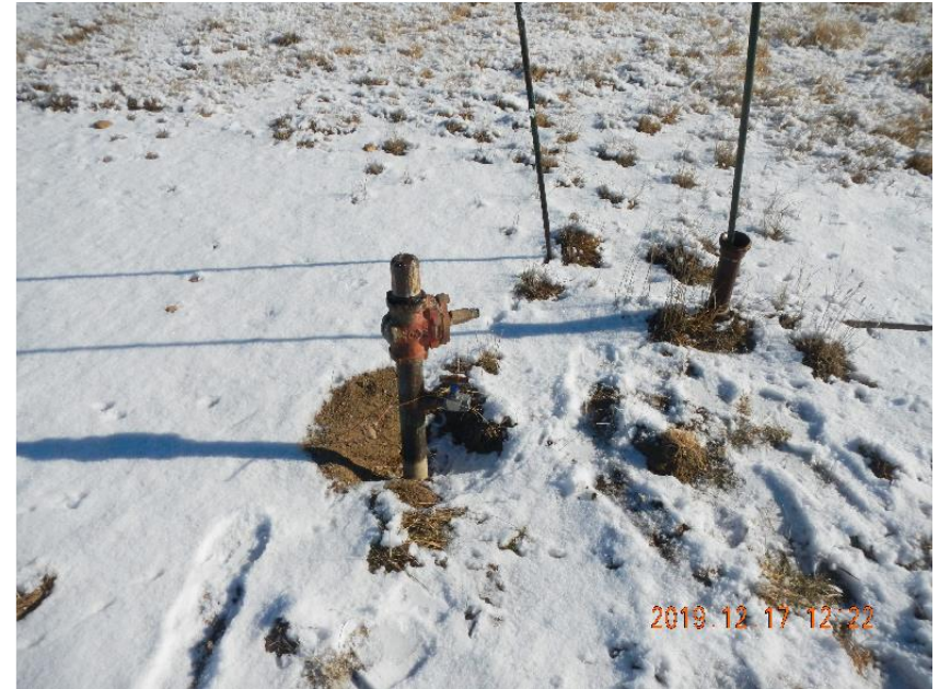
Photo 2: Wellhead and riser..
