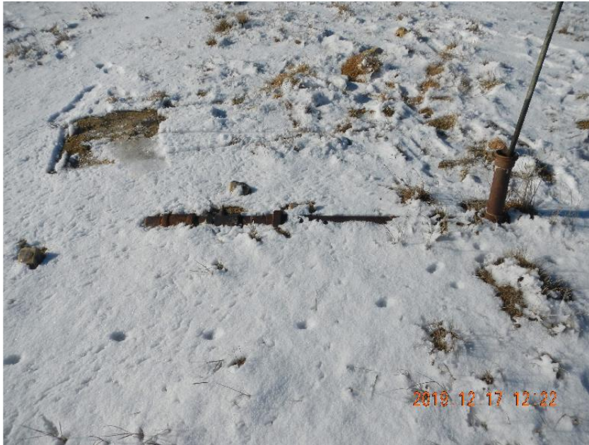
Photo 3: Wellhead and additional flow line.
