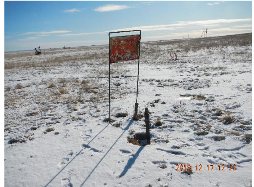
Photo 8: Wellhead and sign.
