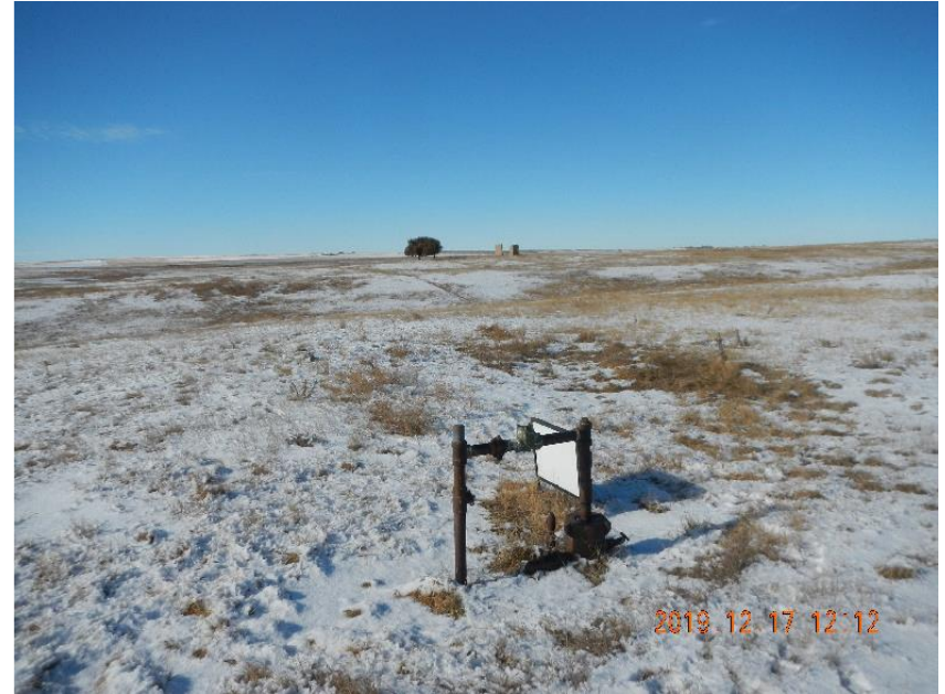
Photo 4: View of wellhead location.
