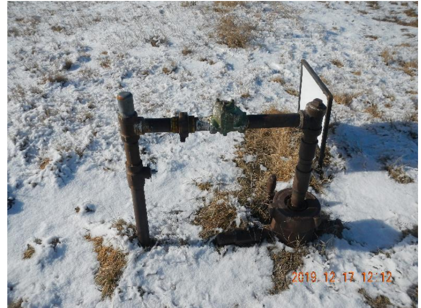
Photo 2: Wellhead and riser.
