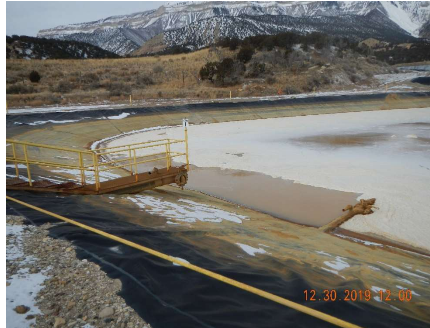
Photo #12 – Flowlines penetrating the liner on the south side of the pit.
