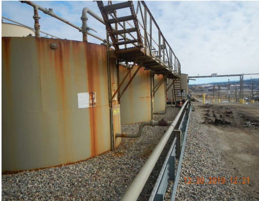
Photo #29 – Rusting three smaller steel ASTs.
