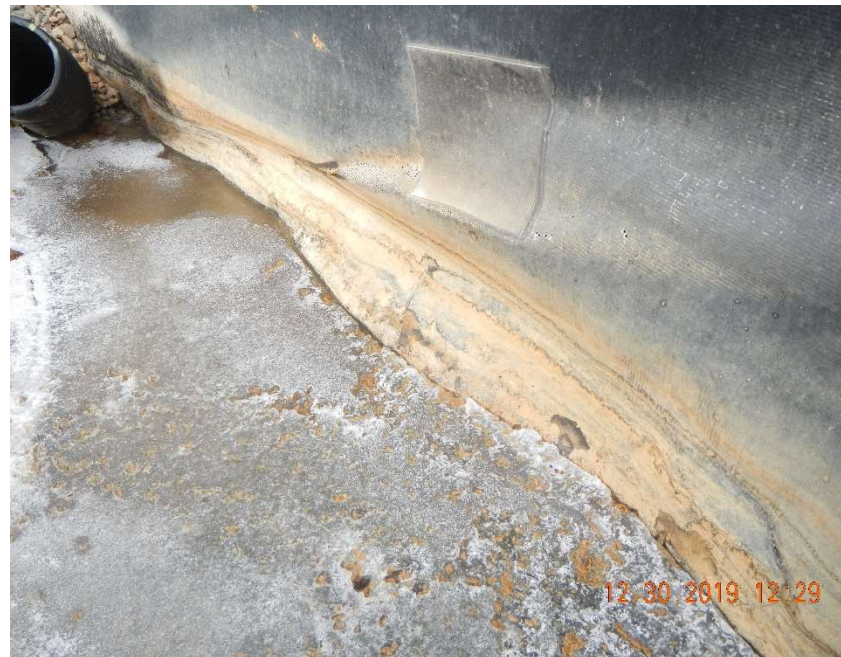
Photo #36 - Secondary containment liner in disrepair.
