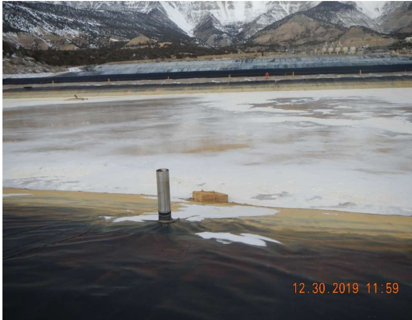
Photo #15 – Concrete anchor resting directly on the pit liner (south side).
