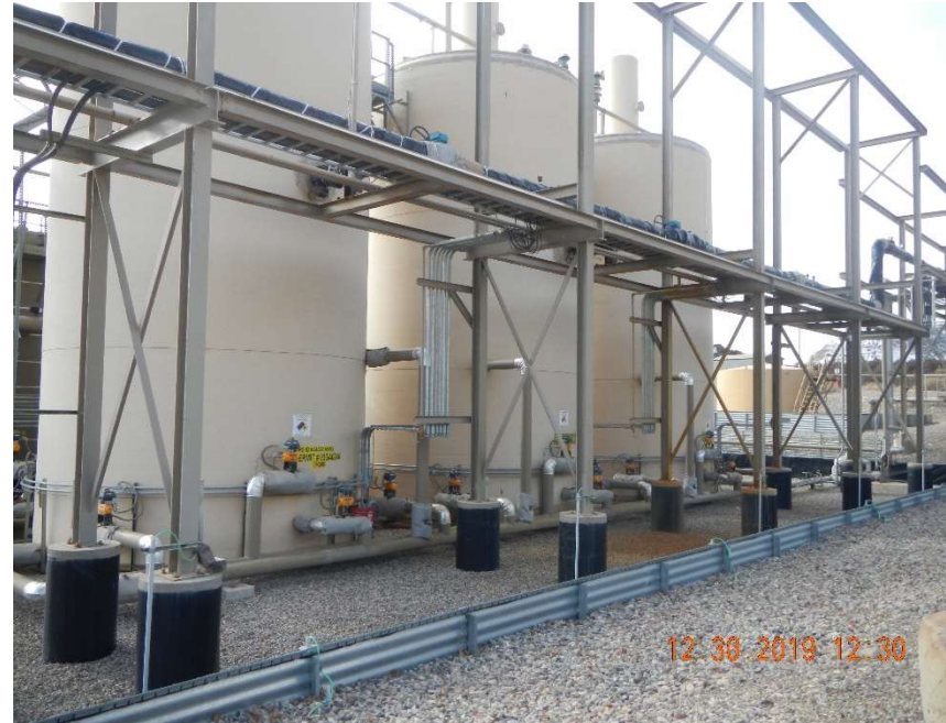
Photo #38 – Three Produced Water steel ASTs.
