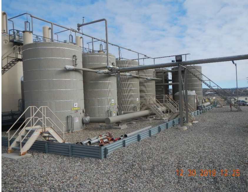
Photo #33 – Six Produced Water steel ASTs and the one 3000 gallon Water Clarification Agent steel AST.
