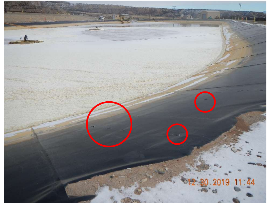
Photo #2 – Various size patches on the pit liner (Red circles).
