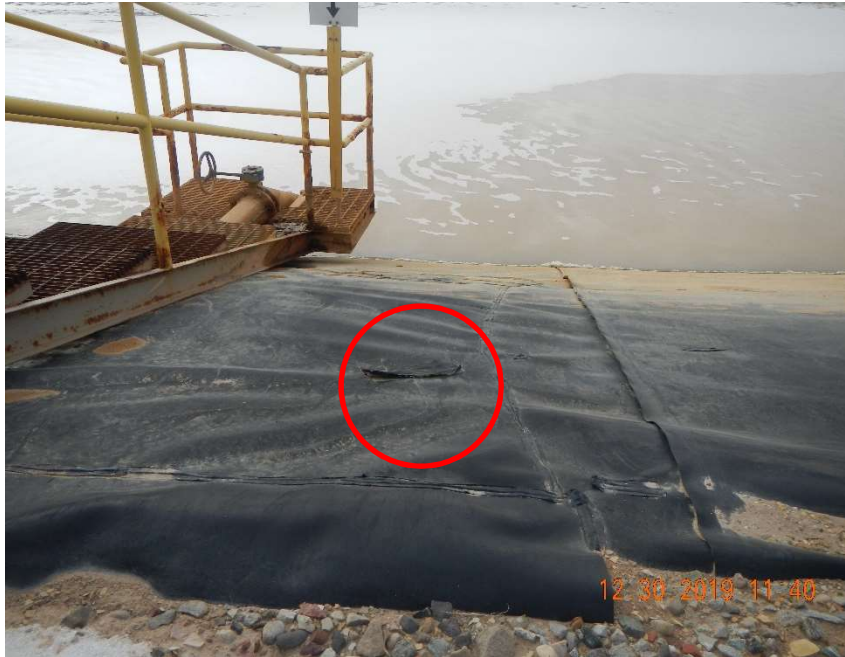
Photo #3 – Patch in disrepair on the northeast corner of the pit liner (Red circle) and a flowline penetrating the liner.
