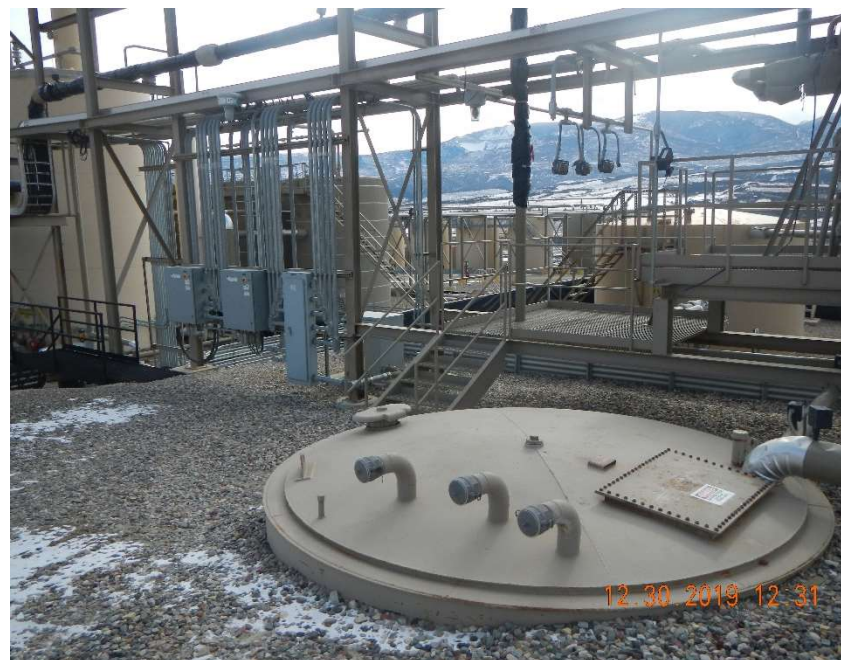
Photo #42 – Partially buried steel AST located north of TK 500.
