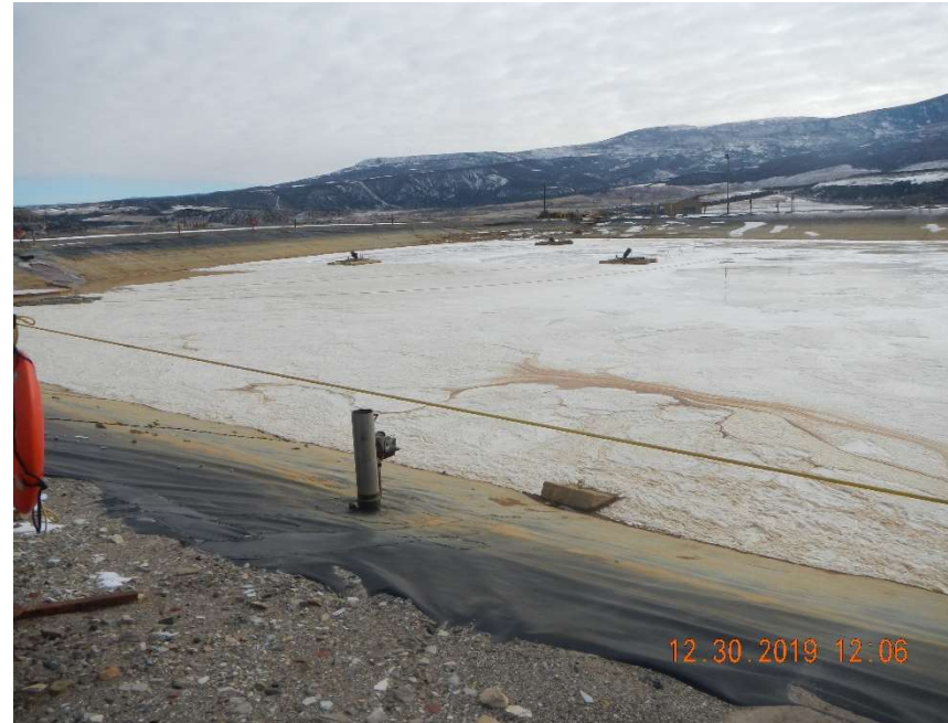
Photo #16 - Concrete anchor resting directly on the pit liner (north side).
