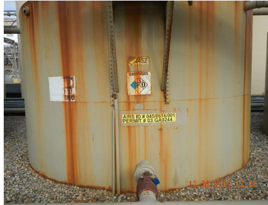
Photo #30 – One of the three rusting steel ASTs missing name of operator, operator emergency contact number and tank capacity.
