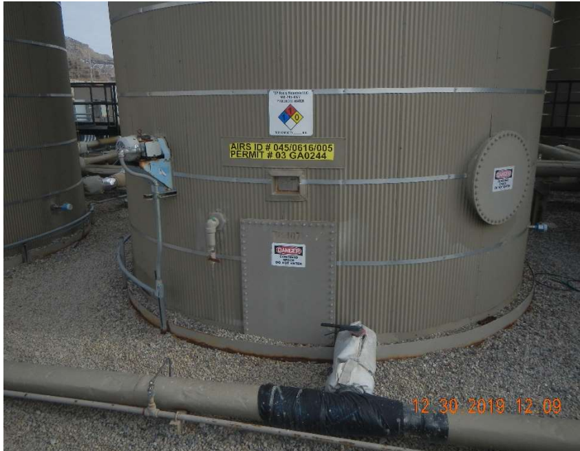
Photo #23 – One of the nine steel ASTs missing the tank capacity label.
