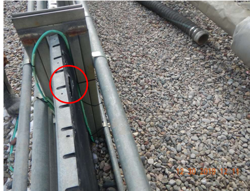
Photo #28 – 2-inch hole in the tank battery secondary containment liner (Red circle).
