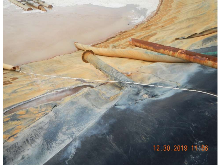
Photo #8 – Flowline penetrating the liner on the east side of the pit.
