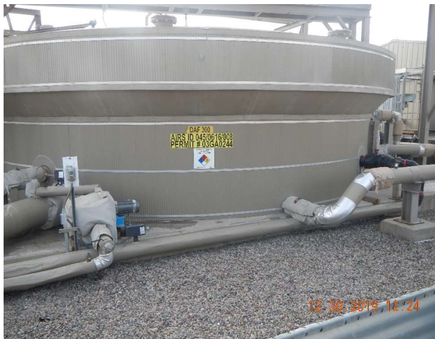
Photo #41 – DAF 300 missing capacity label.
