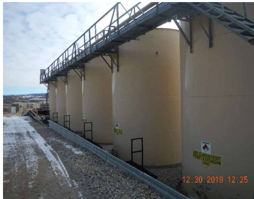
Photo #32 – Six Condensate steel ASTs.
