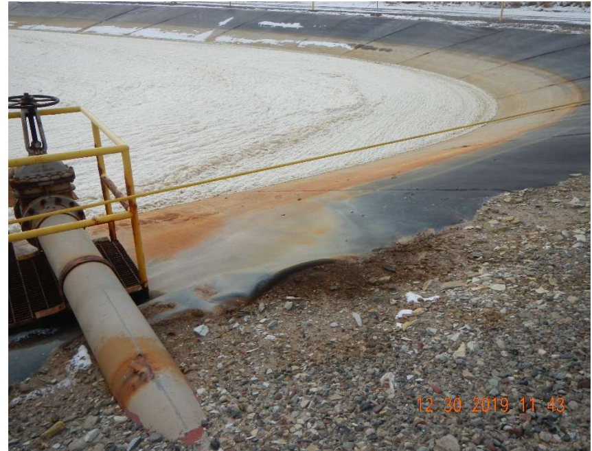
Photo #6 – Impacted soil located on the north side of the pit and staining on the pit liner.
