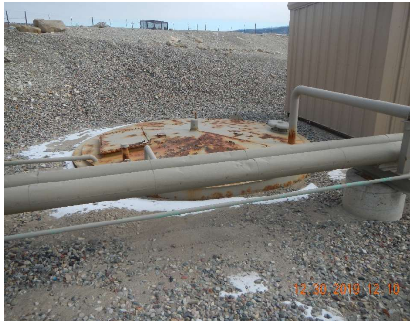
Photo #43 – Partially buried steel AST located north of the lower tank battery.
