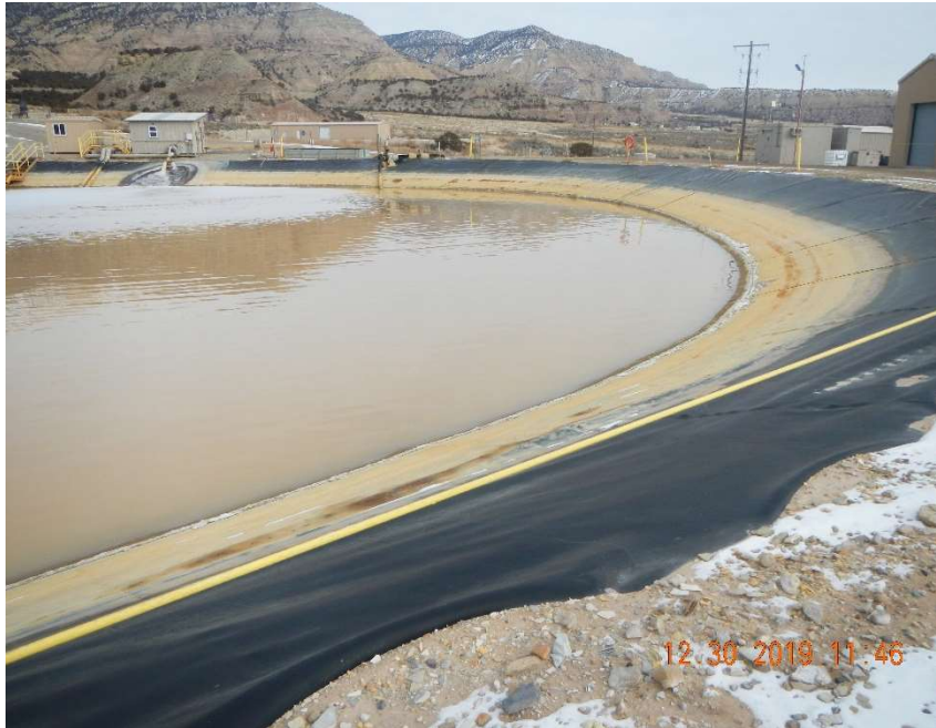
Photo #5 – Four feet of freeboard and staining on the pit liner.
