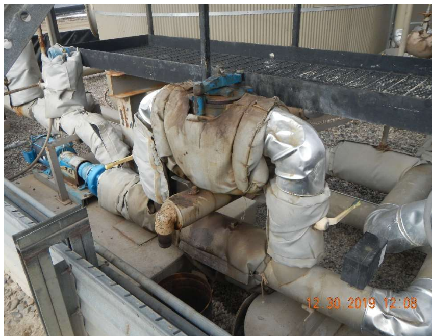
Photo #25 – Five gallon bucket containing hydrocarbons beneath a valve.
