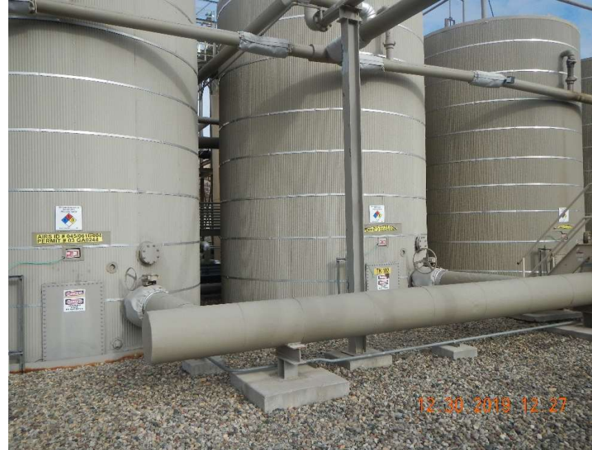
Photo #34 – Three out of the six Produced Water steel ASTs that are missing capacity labels.
