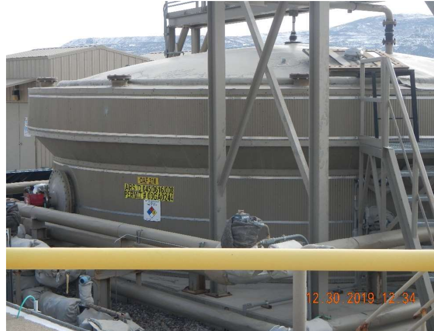
Photo #40 – DAF 310 missing capacity label.
