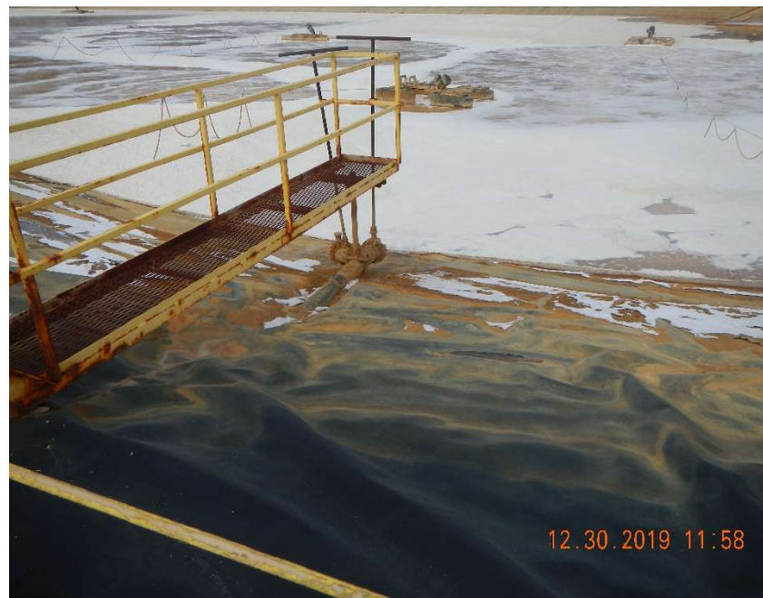
Photo #10 – Flowline penetrating the liner on the south side of the pit.
