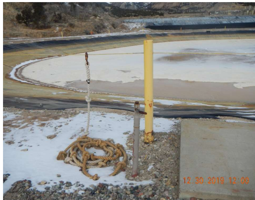
Photo #14 – Unmarked riser on the southwest corner of the pit.
