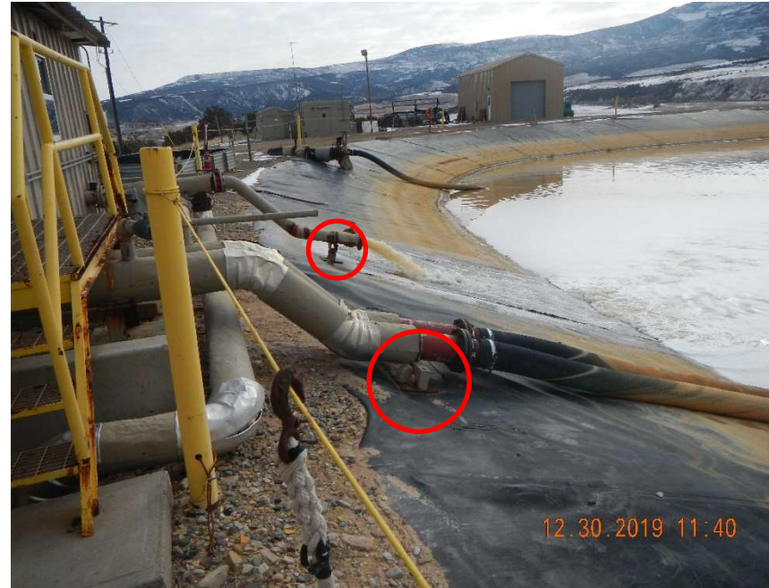
Photo #4 – Metal flowline supports resting directly on the pit liner (Red circles) and staining on the pit liner.
