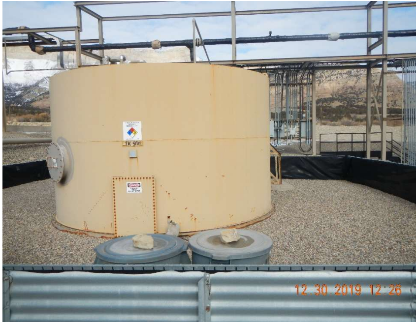
Photo #39 – TK 500 missing capacity label.
