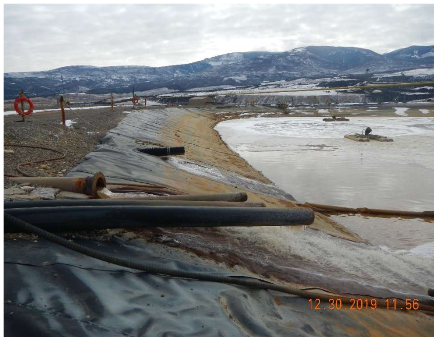
Photo #9 – Flowline penetrating the liner on the east side of the pit.
