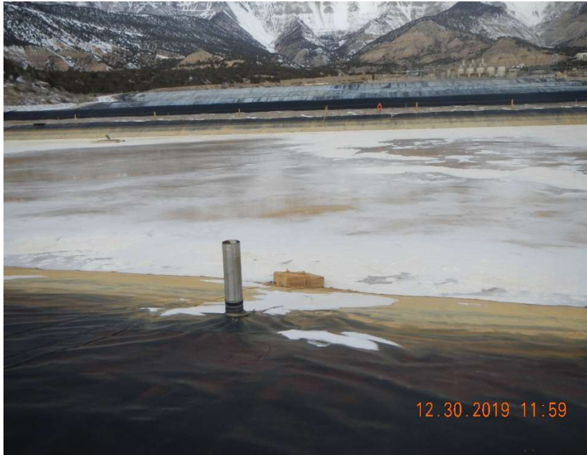
Photo #11 - Flowline penetrating the liner on the south side of the pit.
