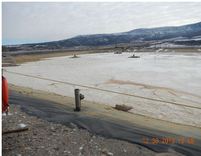
Photo #13 – Flowline penetrating the liner on the north side of the pit.
