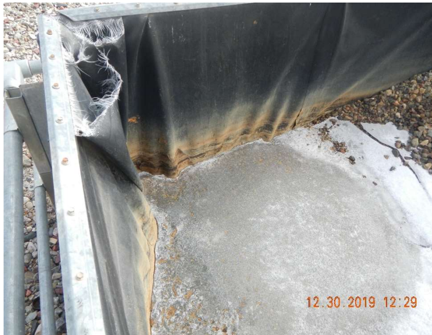
Photo #35 – Secondary containment liner in disrepair.
