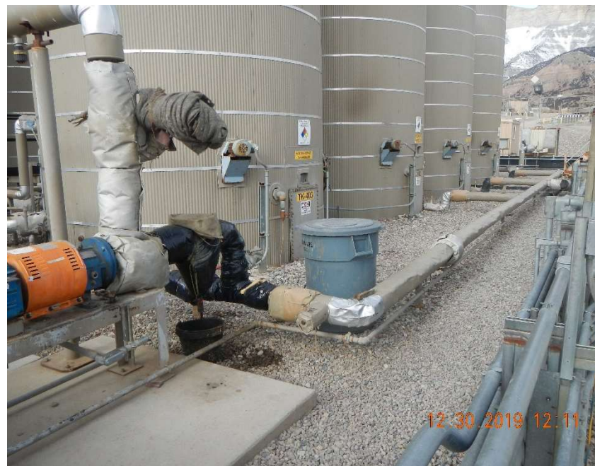
Photo #26 - Five gallon bucket containing hydrocarbons and impacted gravel beneath a valve.
