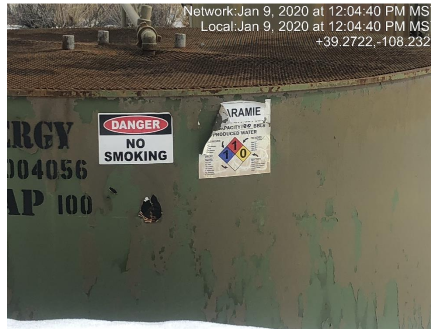
Photo #0376 NFPA label weathered and peeling off tank.
