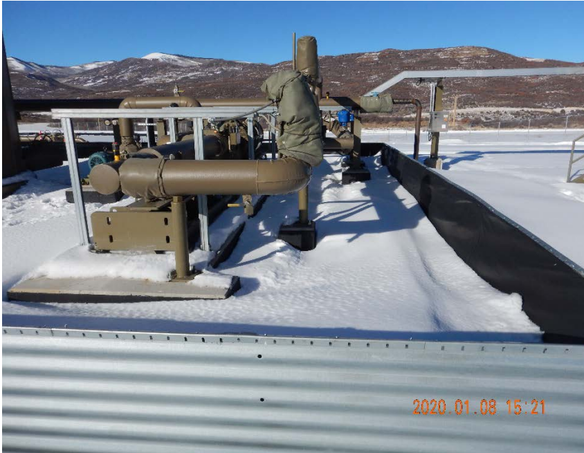
Photo #5 – View of east end of tank battery secondary containment. Presence of snow prevented liner inspection. No holes or tears were observed in visible portion of liner.
