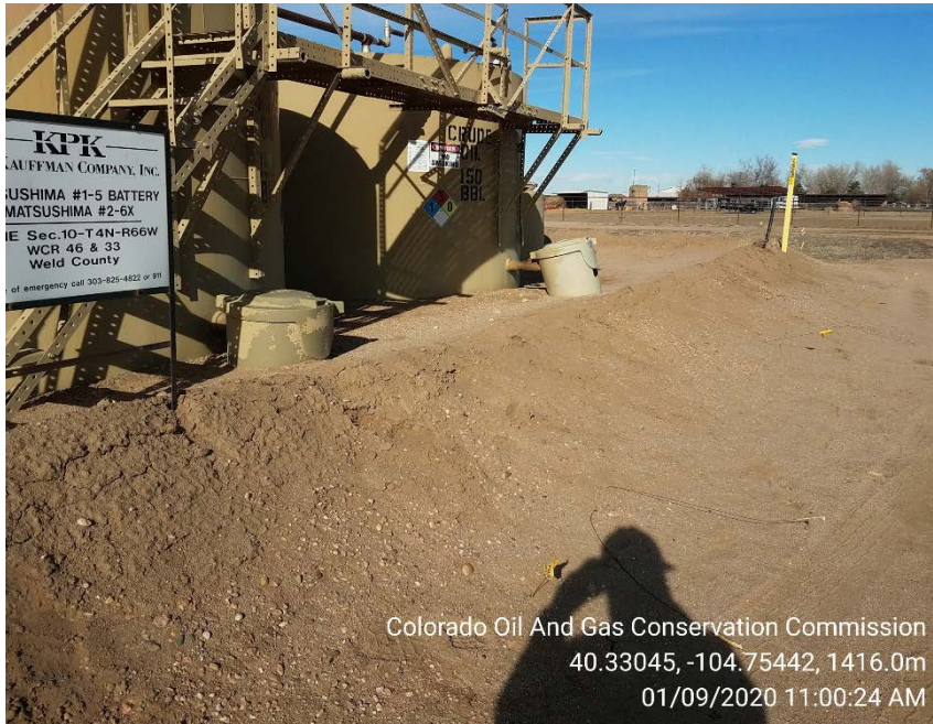
Crude oil tank berm
