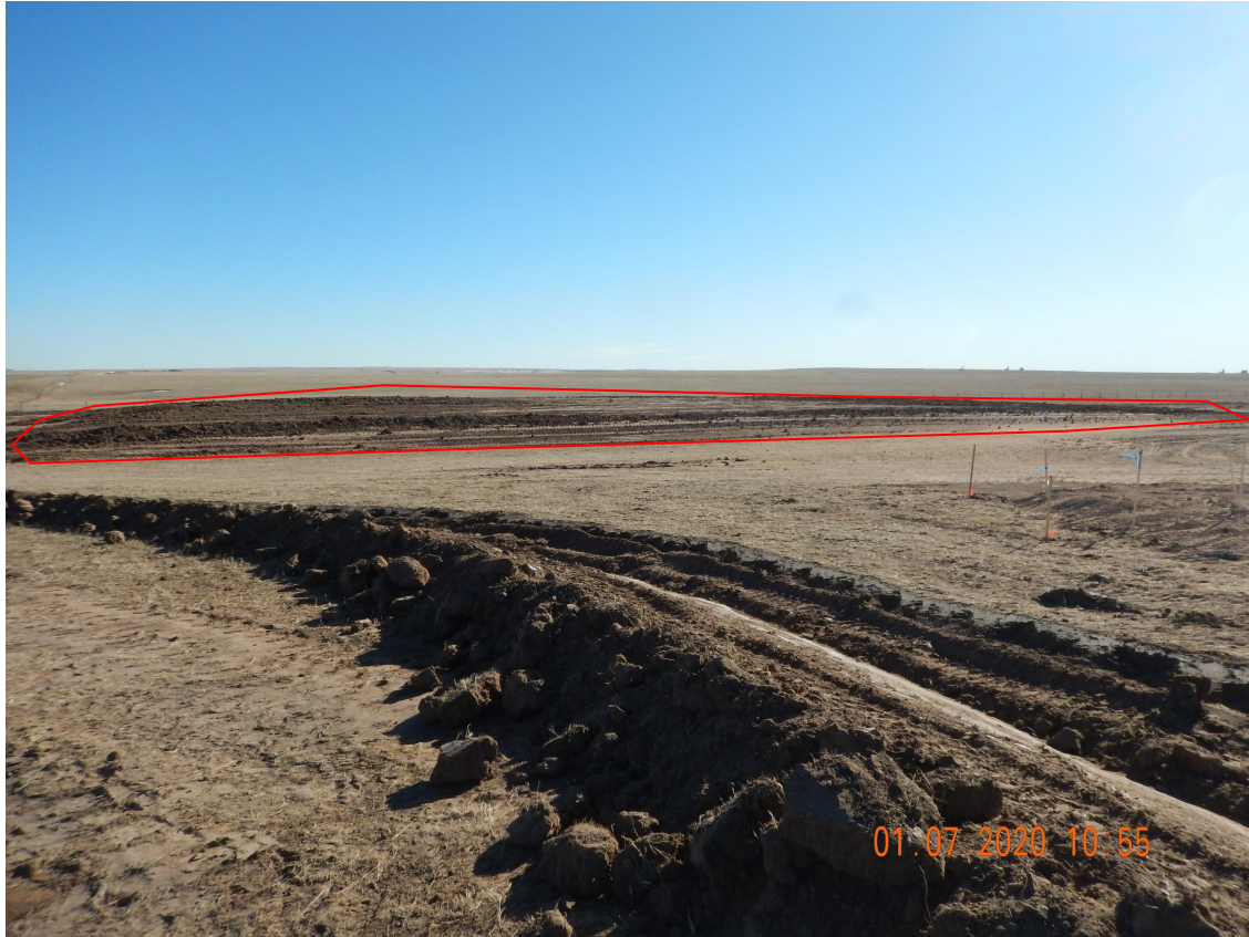
Photo 9. Photo taken from the northern perimeter of location, facing East. Photo illustrates the topsoil stockpile which is being stored along the northeastern portion of the location (highlighted in red).
