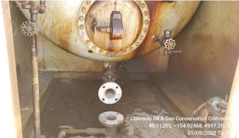
**Photo 7 stained soil inside FWKO housing.**
