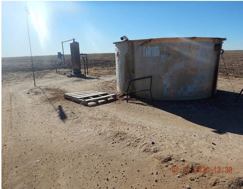
View of facility/ battery. Earthen berms have eroded; inadequate berm capacity. Trash (pallet) on location.
