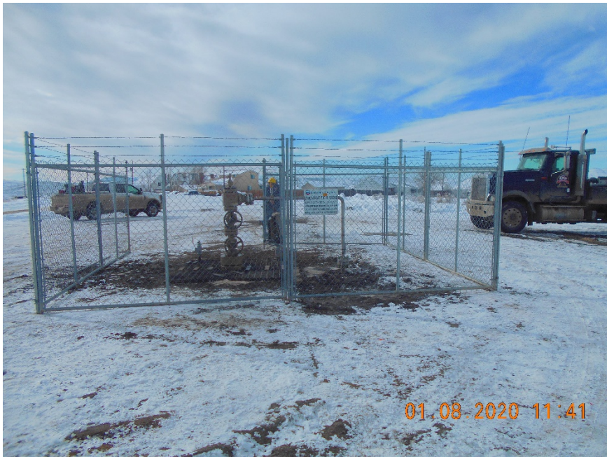
Injection wellhead.
