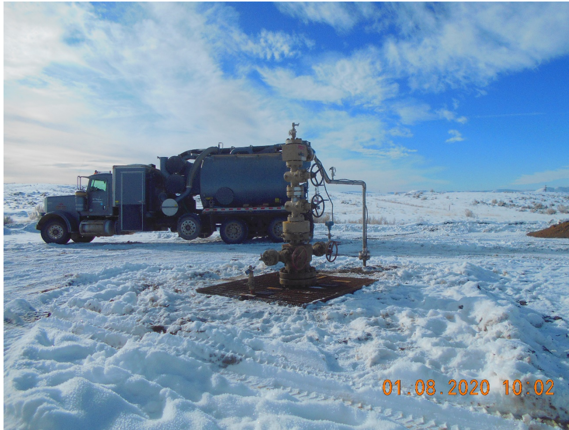
Injection Wellhead
