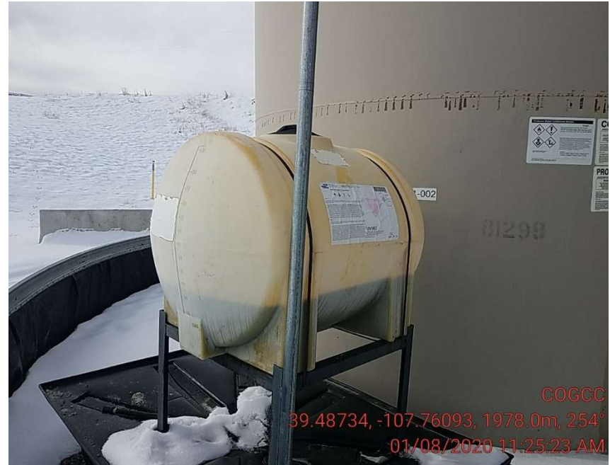
Tank has signage
