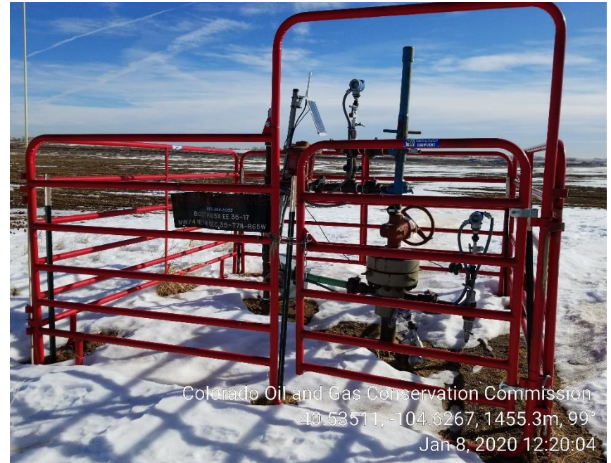
Photo 2: Wellhead; appears weeds are removed (snow covering area)
