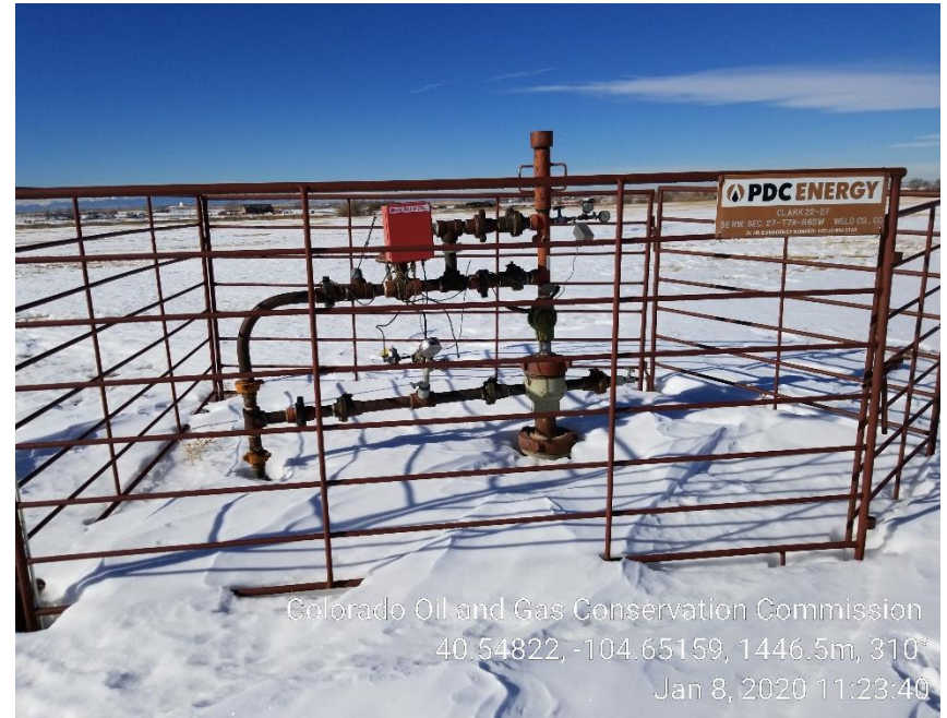
Photo 2: Wellhead; appears weeds have been removed (Snow covering area)
